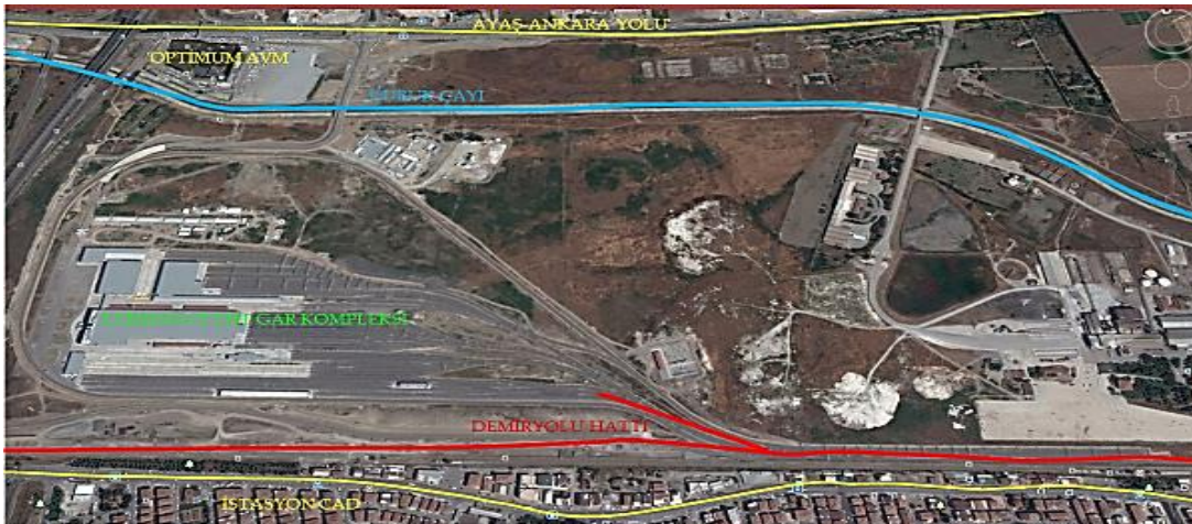
Figure 2.1. Railway Maintenance Complex in Etimesgut-Ankara
