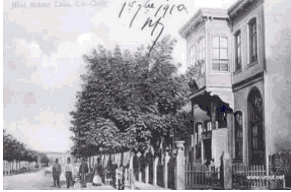
Figure 3. 9. Madam Tadia Hotel in the Railway Station Area 45
