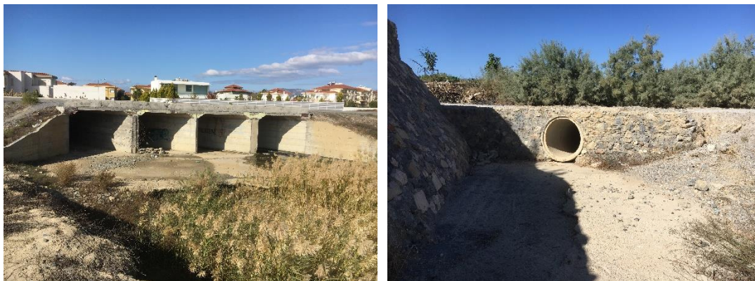
Figure 5.13. Example of bridge and culvert in the study area
