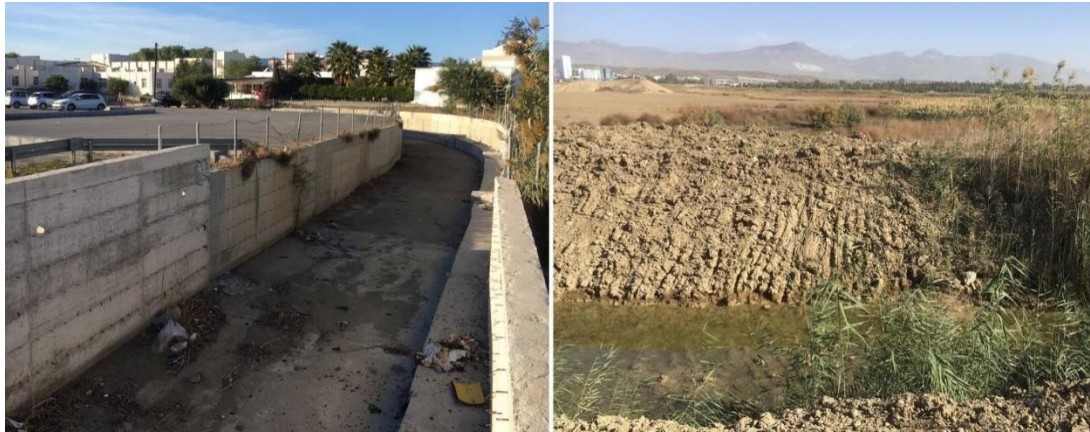
Figure 4.12. Examples for smooth and eroded channels
