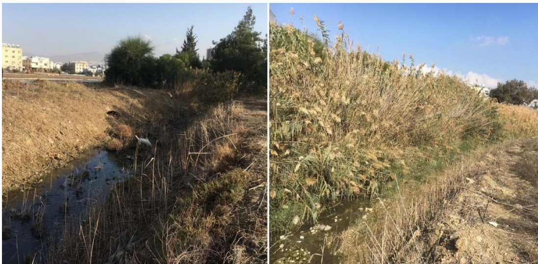
Figure 4.13. Examples for small and very large amount of vegetation in the creeks
