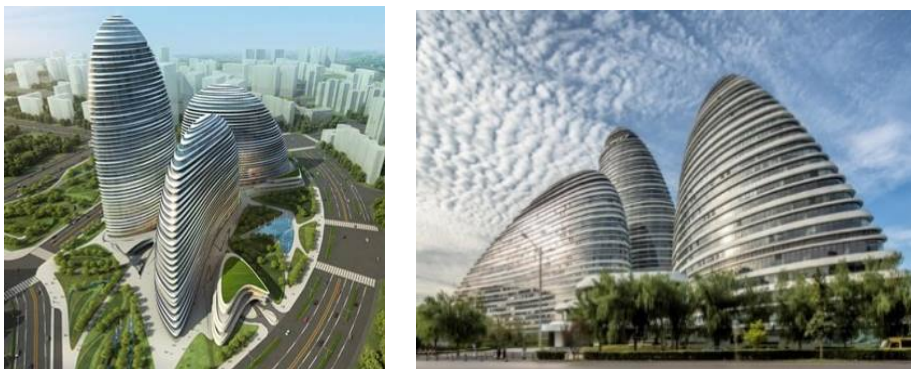
Figure 5. Wangjing Soho, Architect: Zaha Hadid, 2011-2014
