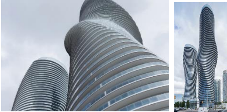
Figure 9. Absolute Towers, Ontario, Canada, MAD Architects, 2012
