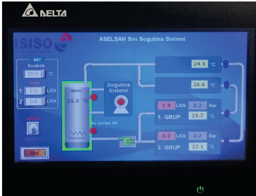
Figure 3.5: User Interface of the custom liquid control unit
