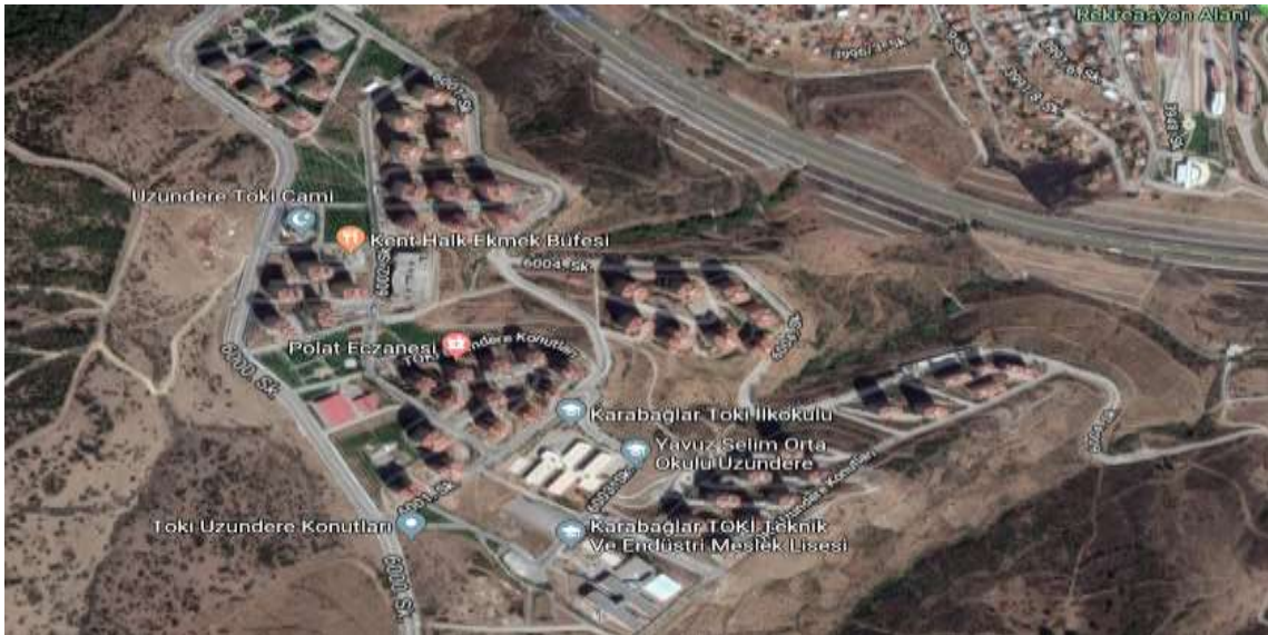
Figure 2: The Distribution of Buildings in TOKİ Uzundere (Google Maps, 2018)
