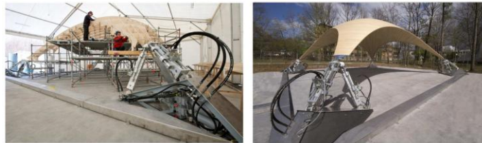
Figure 3.3. Retractable adaptive shell roof structure with hydraulic system, Bosch Rexroth Company
