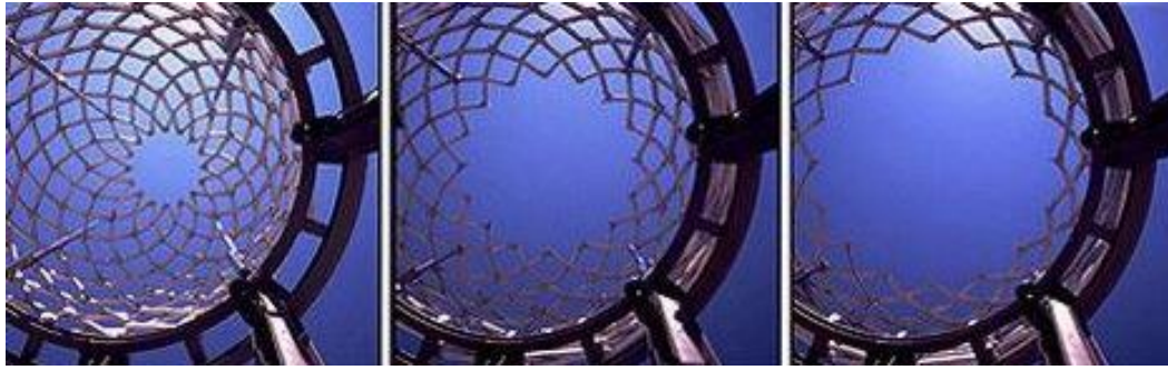
Figure 3.13. In 1994, Iris Dome is designed by Hoberman with angulated scissors mechanism
