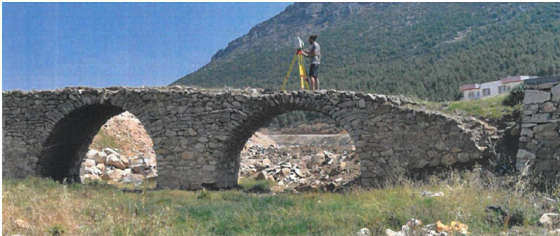
Figure 3.1. Onaç Masonry Bridge (YAVUZ MİMARLIK, 2017)
