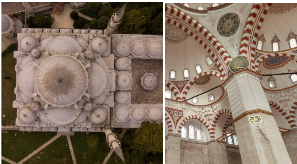
Figure 3.9. Internal and external complex geometry of Şehzade mosque
