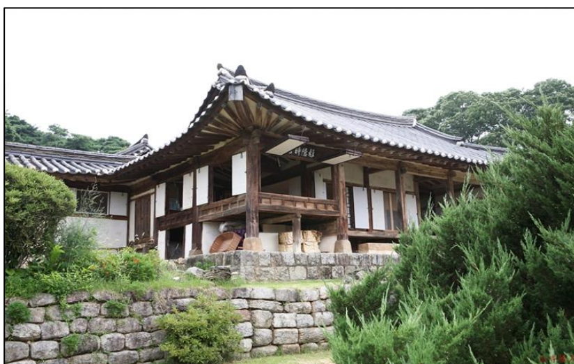
Figure 83 Low Dam of Inner Room of Yunjung House in Nonsan of Chungnam
