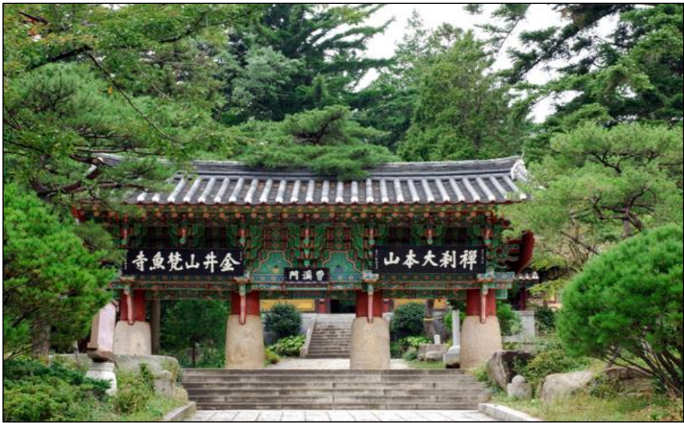
Figure 22 Short and White Columns Being Used in the Beomesa Temple in Busan
