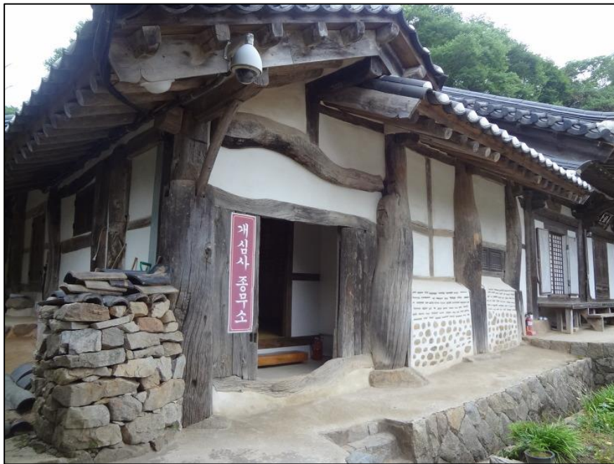
Figure 34 Irregular Shape of Wooden Columns of Gesimsa Yosache Temple Built in 1350
