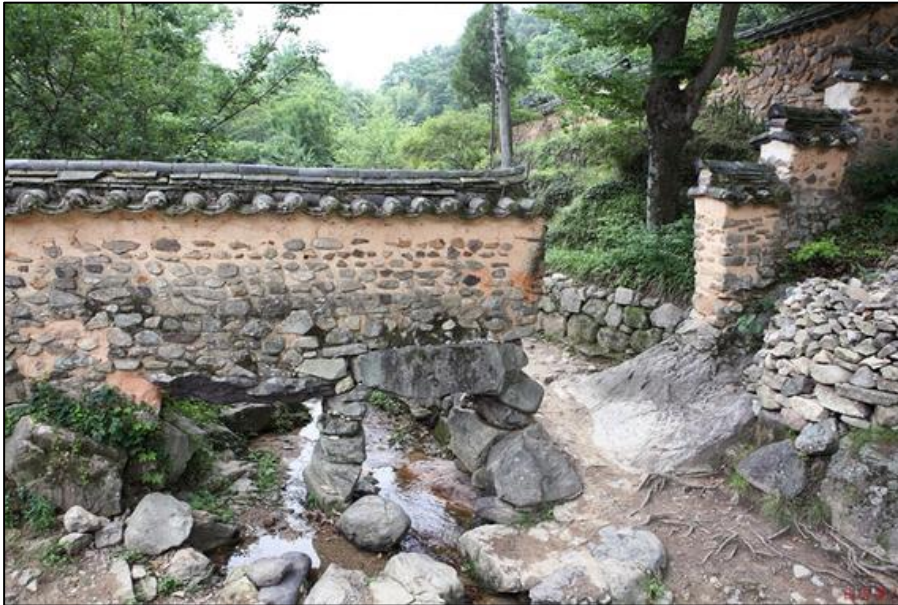
Figure 84 Cut Dam of Sosewon in Yehang of Jeonnam
