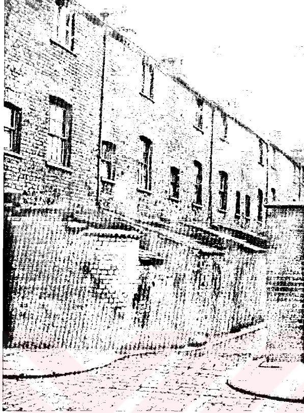
Figure 6. An example of terrace houses in Manchester (Burnett, 1978: 120).
