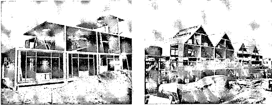
Figure 40. Molenvliet housing complex. Left: the “support”; Right: the preparation of “in-fill kits” (Hatch, 1984: 333).
