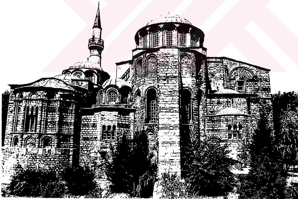
Illustration 8: East facade, present state of the edifice.
