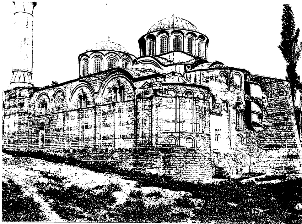
Illustration 9: Southeast view, present state of the edifice.
