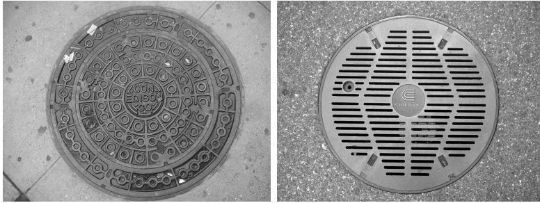
Figure 4 This is an image of a solid cover (left) and a new vented cover (right). Source: Flickr, photostreams of Nick Sherman and i.follow.
