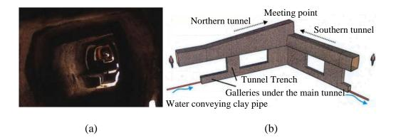
*Figure 2.1.* The Tunnel of Samos (a) Cross Section of the tunnel (Apostol, 2004); (b) A sketch of meeting points of the tunnel boring sections (Angistalis and Kouroumli, 2014)
