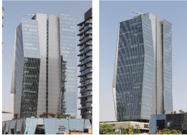
Figure 3.8. Photographs of Next Level
