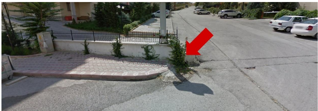
Figure B.5. Ramp on the pavement is obstructed by a tree.
