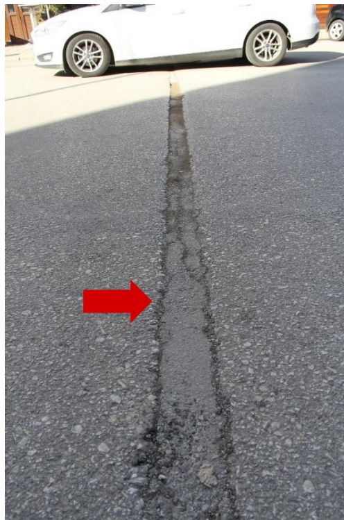
Figure B.9. Fiber-optic Cable Installation board etc.
