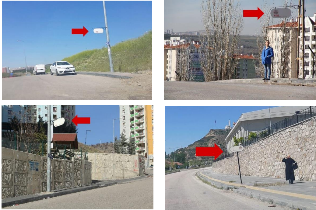
Figure A.1. Transportation facilities lacking shelters, sitting facilities, real-time bus arrival information board etc.
