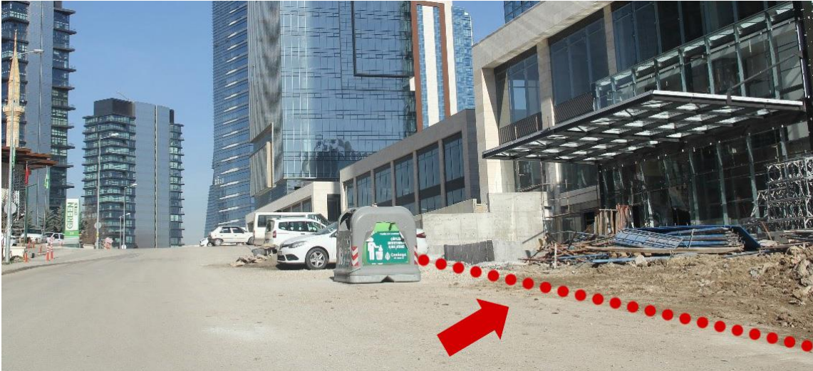
Figure B.6. Lack of pavement around construction sites
