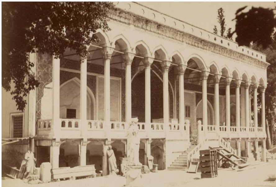
Figure 4 The Tiled Kiosk after renovation
