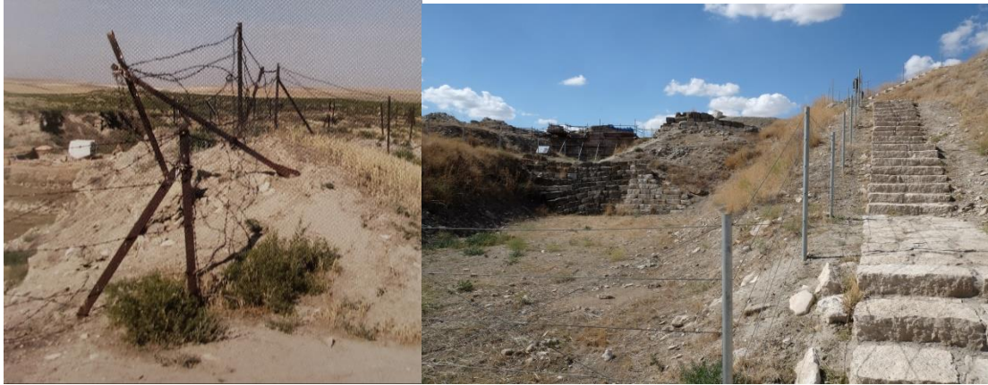
Figure 35 The old rusted fence along the visitor circuit before 2009
