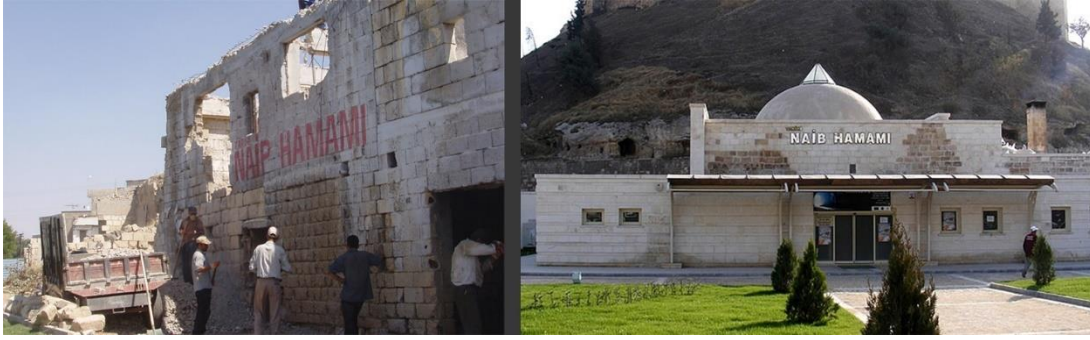
Figure 4.25. Renovation of Naib Hot Bath (Source: Kutay İnşaat, 2019)
