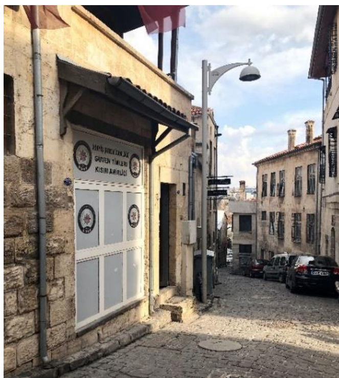
Figure 4.53. Recently Opened Police Station for Security Problems (Photo taken by the author, 2019)
