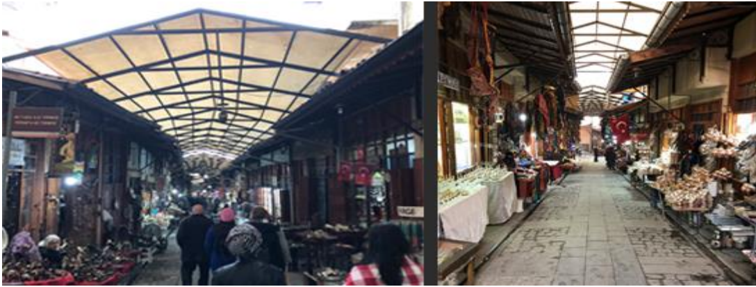
Figure 4.37. Roofing the Bakırcılar Bazaar and Street Arrangements which Enable Protection of the Products (Photos taken by the author, 2019)
