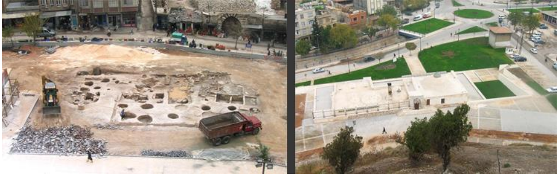
Figure 4.17. Landscape Project Implementation of the Castle (Source: Kutay İnşaat, 2019)
