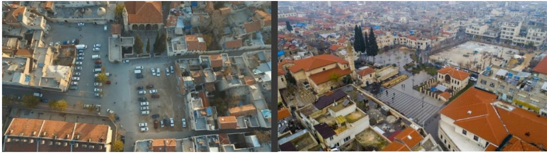
Figure 4.61. Şih Square, Before the Interventions (left) and After the Implementations (right) (Source: Şahinbey Municipality Website, 2019)
