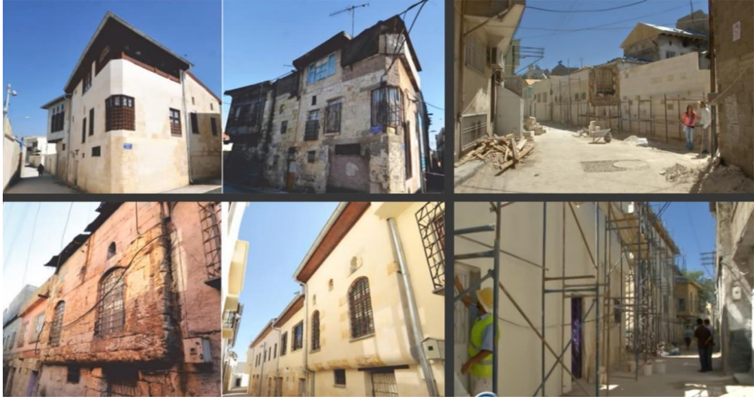
Figure 4.58. Façade Restorations and Street Rehabilitations in Kepenek Neighborhood (Şahinbey Belediyesi, 2013)
