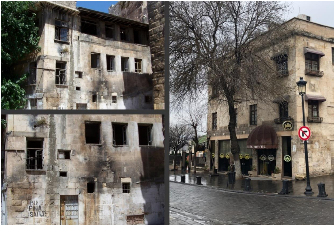
Figure 4.26. Renovation of Boutique Hotel (Source: Kutay İnşaat, 2019)
