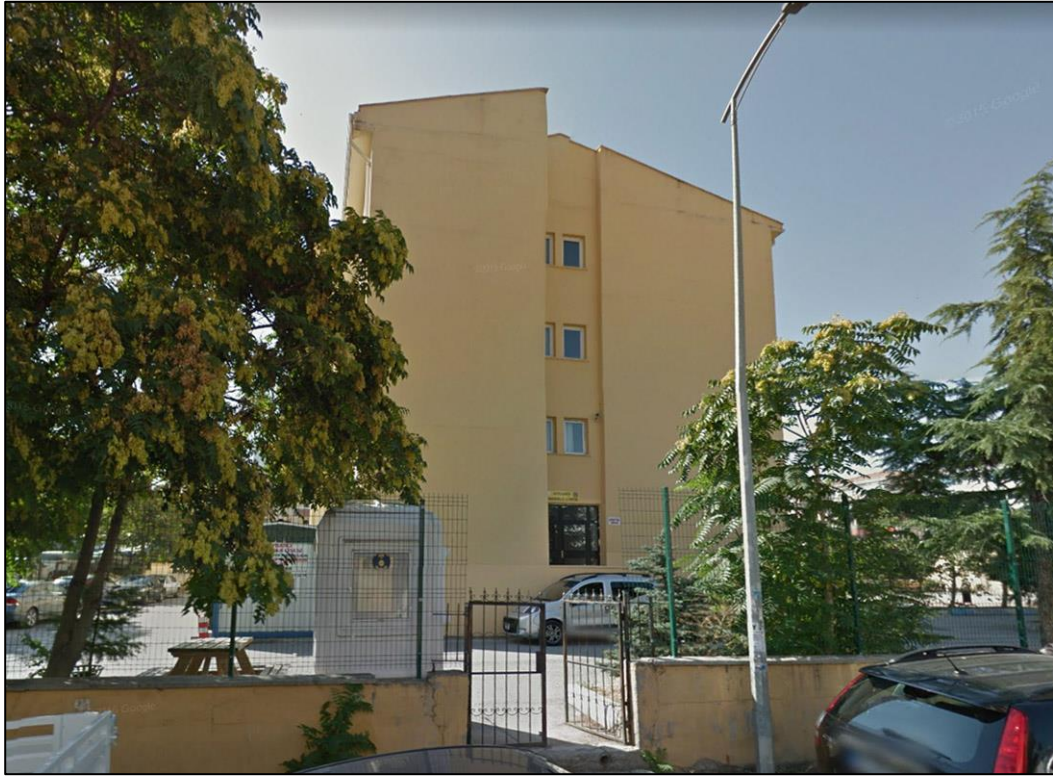
Figure 3.8. North façade of the school building
