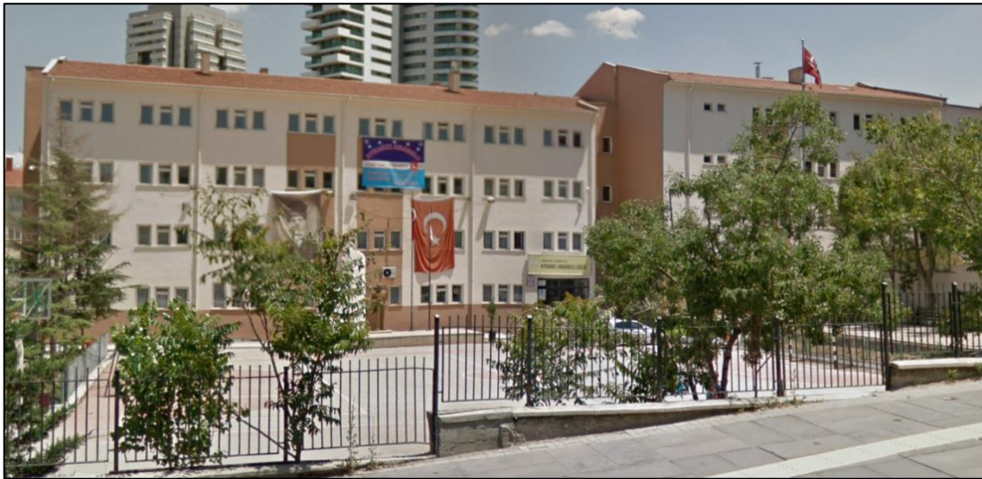
Figure 3.7. West façade of Ayrancı Anatolian High School in Ankara
