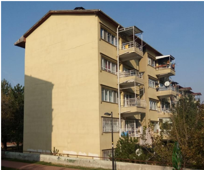
Figure 3.4. Photo showing the front and side façades of one of the first case study apartment buildings
