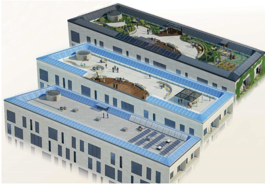
Figure 3.10. PV panel installation, roof design possibilities (Axitecsolar, 2014)
