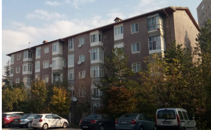
Figure 3.5. Photo showing the rear facade of the first case study apartment buildings
