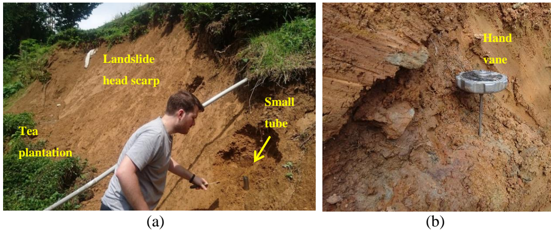
Figure 3.3. Field works at different landslide sites, (a) Intact sampling by small tube insertion at the side scarp of one of the landslides in site 10-1, (b) Field vane test at site 7
