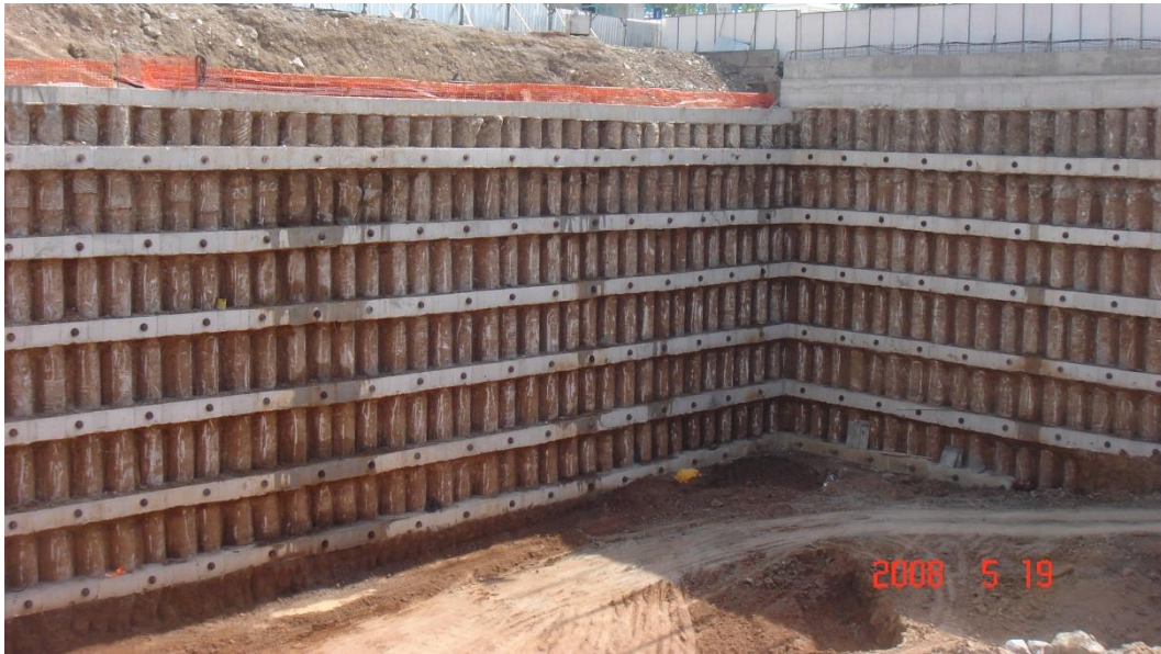
Figure 2.19. Picture from the Deep Excavation Site (Çalışan, 2009)
