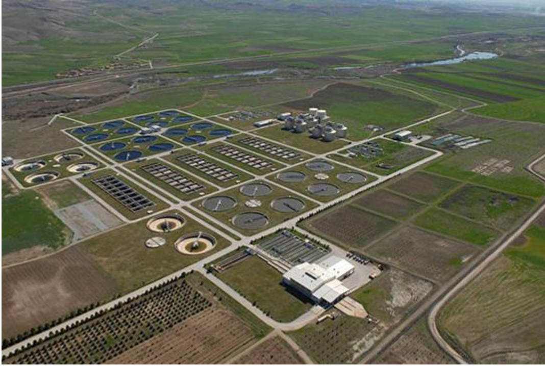
Figure 3-2. Air View of Tatlar Wastewater Treatment Plant (ASKİ Genel Müdürlüğü, 2019)
