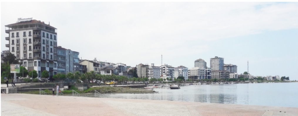
Figure 6.29. Photograph related with facade continuity in Zone 1 (Author's Personal Archive)
