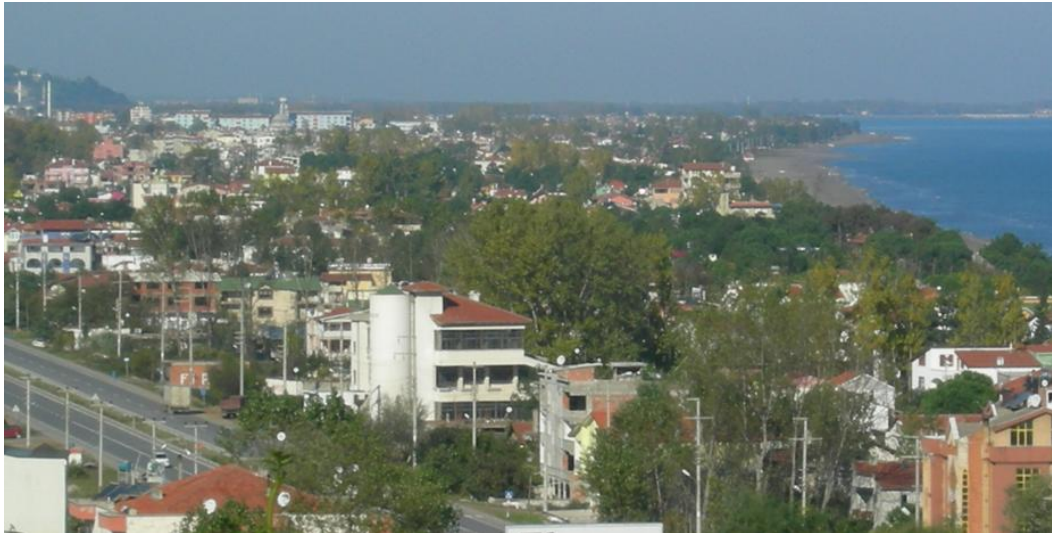
Figure 5.17: New summer houses between Dereköy and Engiz (Yılmaz, 2011, p.12).
