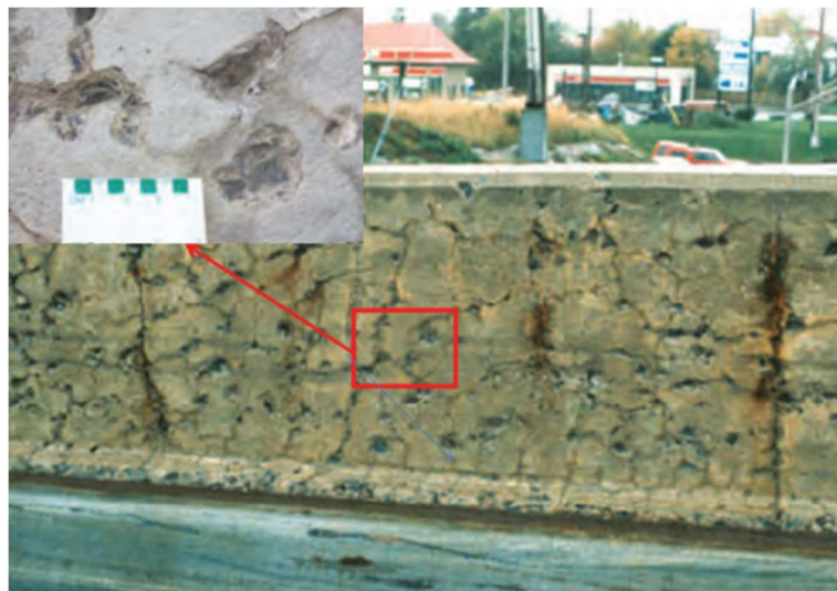
Figure 15. Pop outs in concrete [6]
