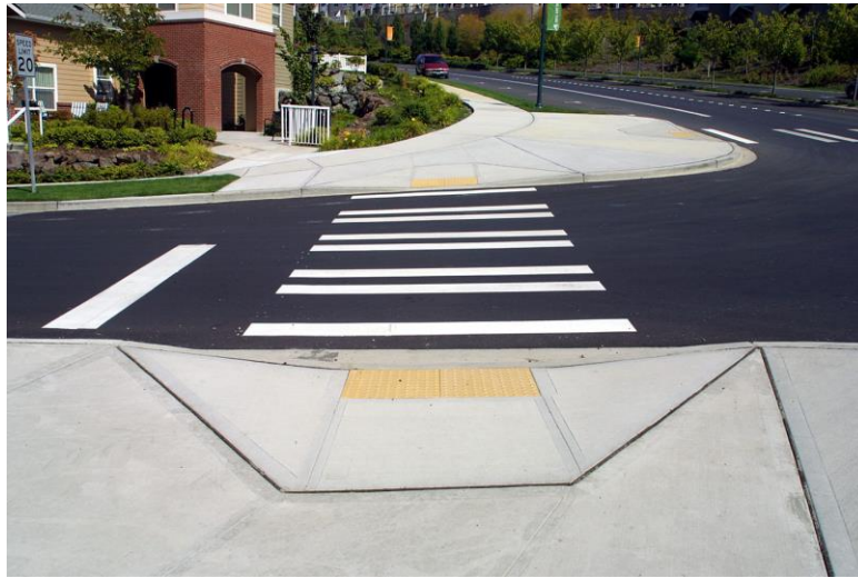
Figure 2-12. Good example of crosswalk (Burden, 2006)
