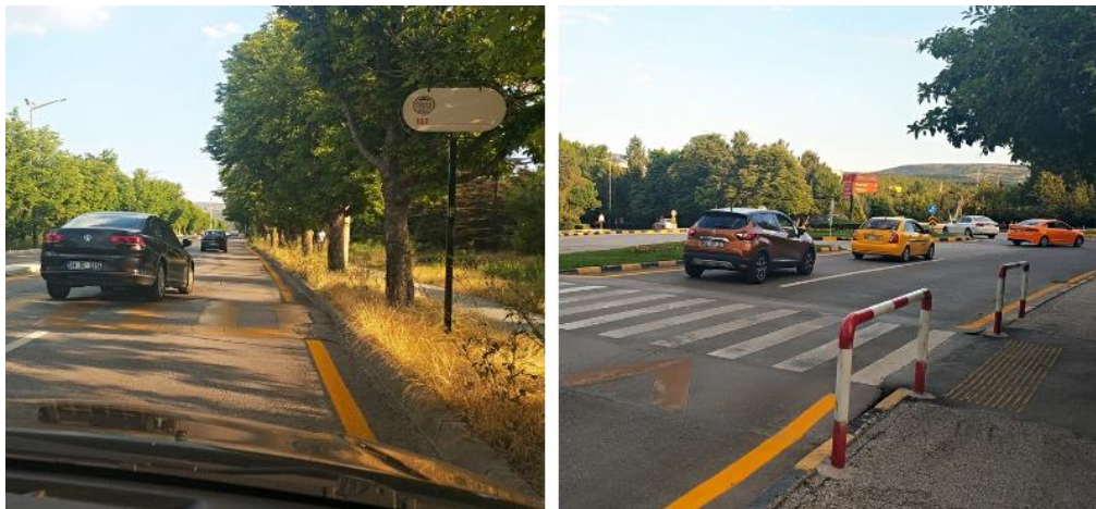
Figure 5-20. Examples of protective barriers in METU campus
