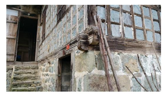
Figure 4.5. Beam joints on Arılı 91
