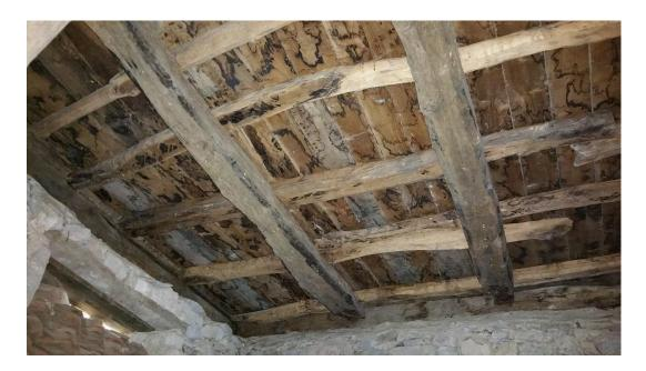
Figure 4.11. Flooring planks of Yukarıhacılar case seen from the ground floor
