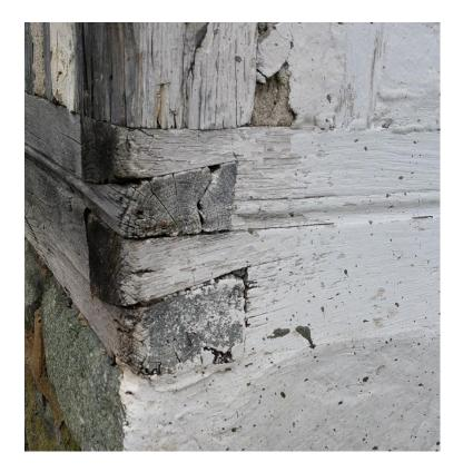
Figure 3.26. Kertme boğaz joint of Dereüstü 28
