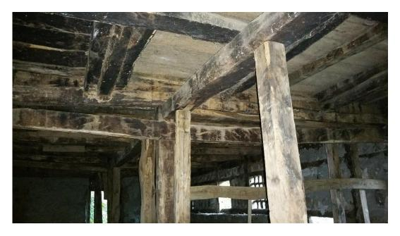
Figure 4.21. Post and beam system in the ground floor supporting first floor
