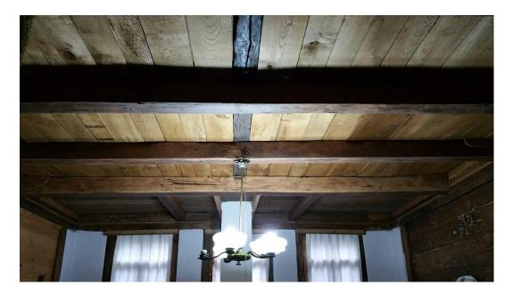
Figure 3.52. Inverted plank ceiling in Dereüstü 20
