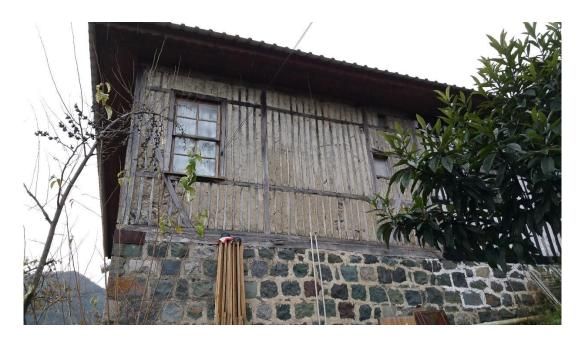
Figure 3.14. Çatma walls of Dereüstü 20
