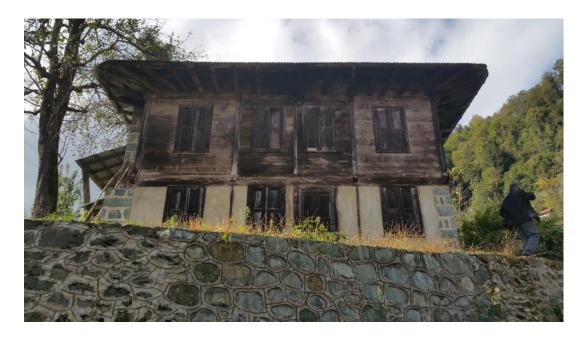
Figure 3.18. Timber infill wall technique in Arılı
