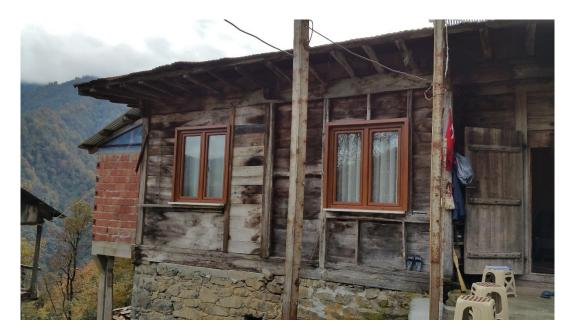
Figure 3.17. Timber infill walls of Arılı 33
