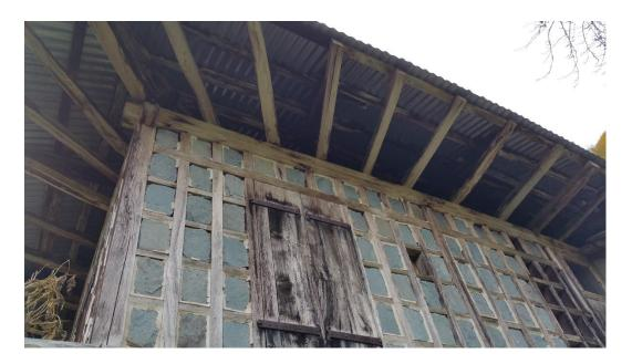
Figure 4.10. Corrugated metal roof covering of Arılı 91
