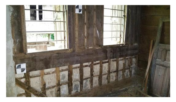
Figure 3.22. Timber plank siding with missing elements in Şenköy 3
