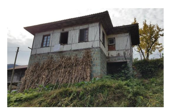
Figure 4.1. Masonry walls of the ground floor and foundation of Arılı 105
