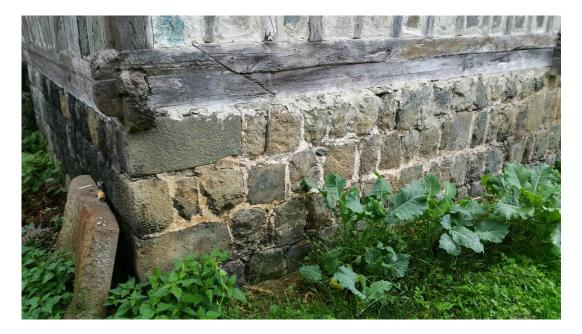
Figure 3.28. Diagonal lengthening details seen on Şenköy 3
