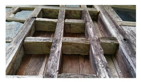
Figure 4.6. Göz dolma technique on Arılı 91
