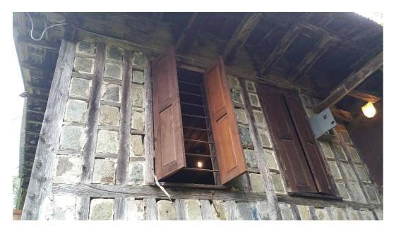
Figure 4.33. Timber shutters and metal guards
