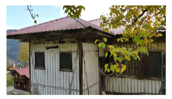
Figure 4.9. Corrugated metal roof covering of Arılı 105
