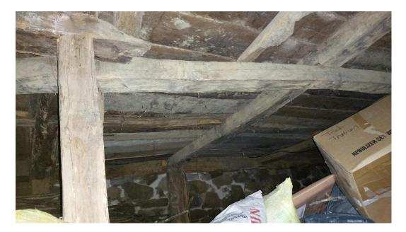
Figure 4.4. Post and beam system in Yolgeçen 80
