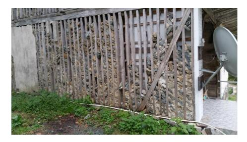
Figure 3.15. Çatma wall skeleton and infill material in Arılı
