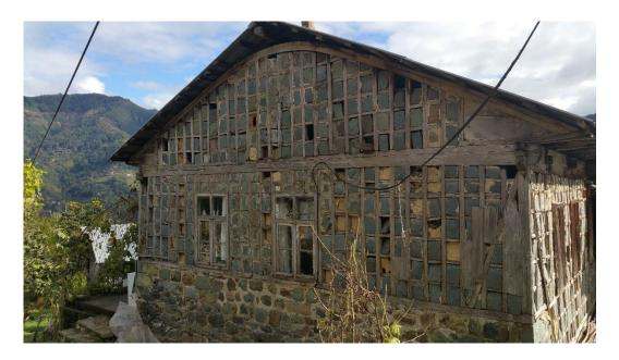
Figure 3.33. A curved sağrıcık gable with removed half hip in Arılı
