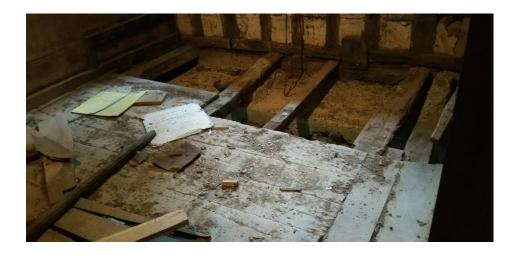
Figure 3.50. Timber plank flooring of Şenköy 3
