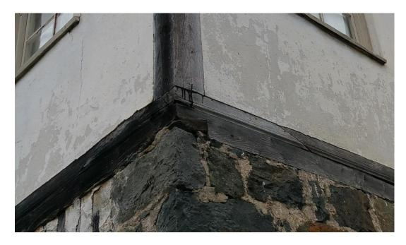
Figure 3.27. Diagonal bonding on Dereüstü 20 with a single timber element that are joined to beams at two sides similarly to the lengthening joint
