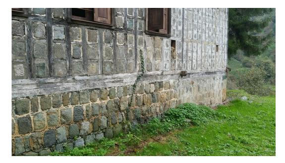
Figure 4.20. Wall plates with kurt boğaz joints
