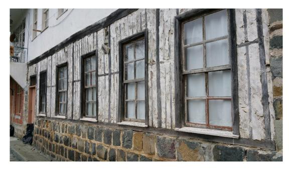
Figure 4.3. Timber frame section of the ground floor walls of Dereüstü 28
