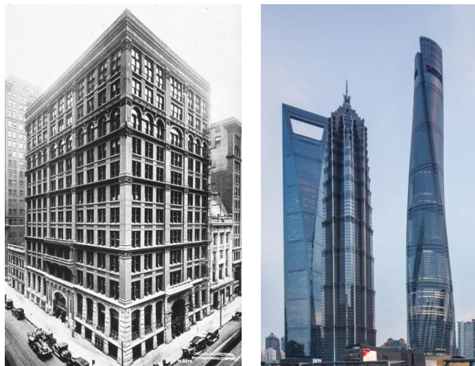
Figure 2.1. (Left) Home Insurance Building (1885) Source: The Skyscraper Center, (Right) Shanghai WFC (2008), Jin Mao Tower (1999), Shanghai Tower (2015) Source: Gensler
