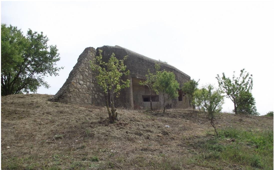
Figure 4.19 Bunker Type 4, openings on front façade, Photographed by the author on 25/04/2019
