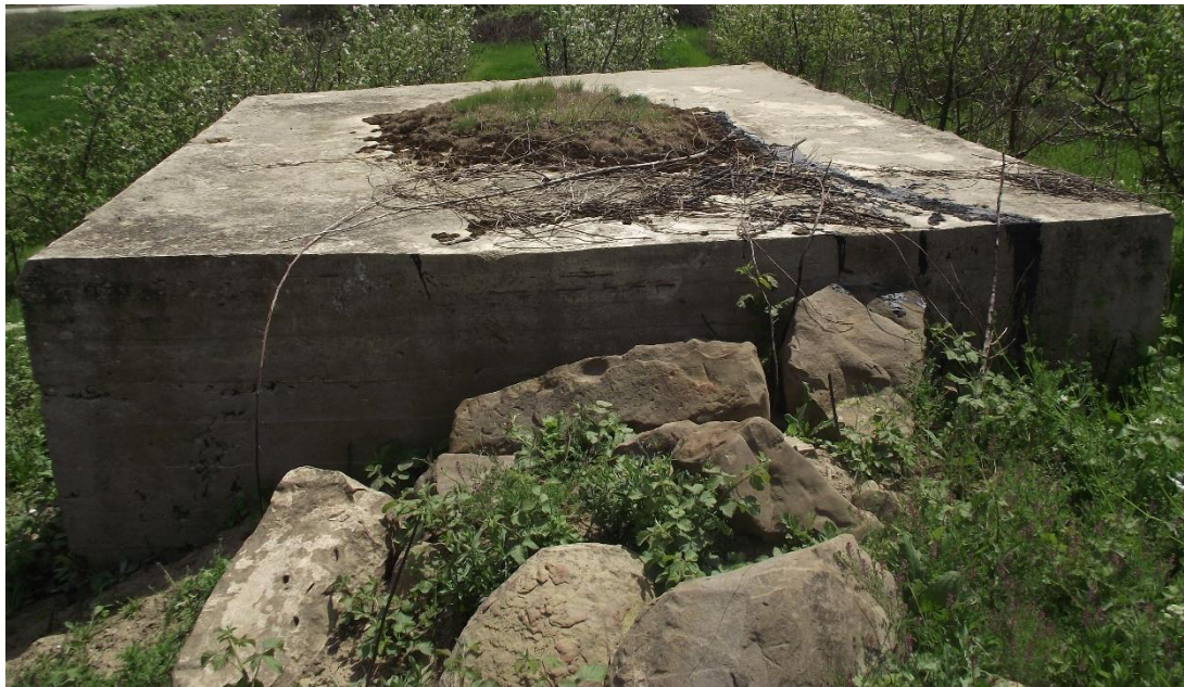
Figure 4.5 Bunker Type 1, side view photo, Photographed by the author on 25/04/2019
