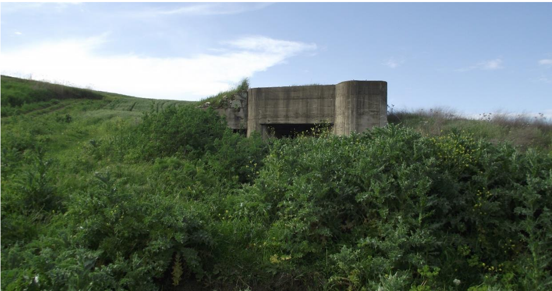
Figure 4.15 Bunker Type 3, openings, Photographed by the author on 02/05/2019
