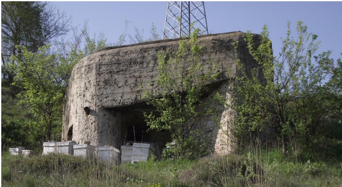
Figure 4.13 Bunker Type 2, with a thick slab, Photographed by the author on 27/04/2019
