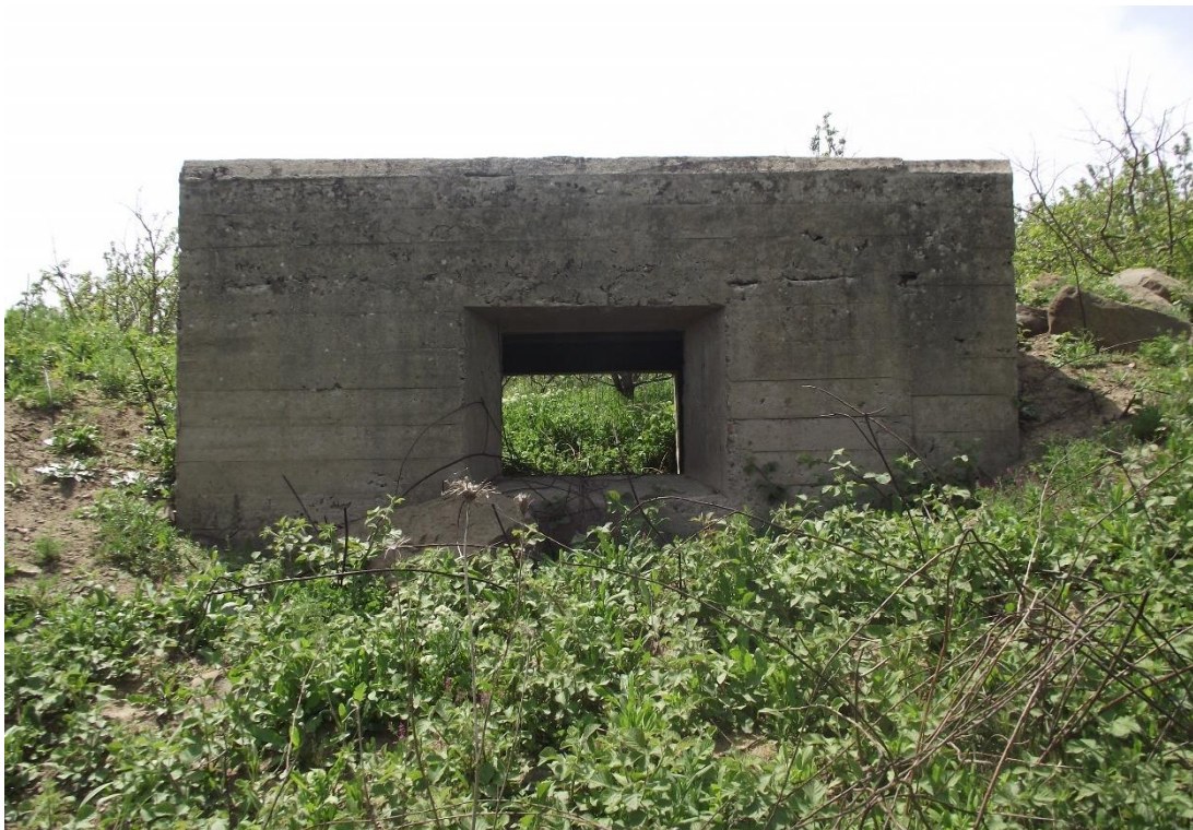
Figure 4.7 Bunker Type 1, front view photo, Photographed by the author on 25/04/2019
