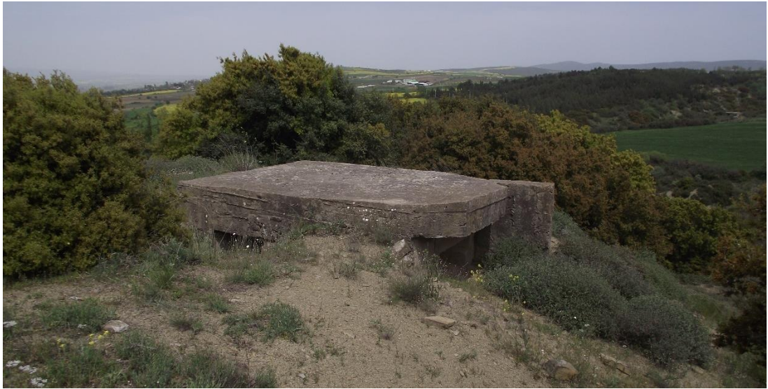
Figure 4.9 Bunker Type 2, side view photo with eaves, extension and side entrance Photographed by the author on 27/04/2019
