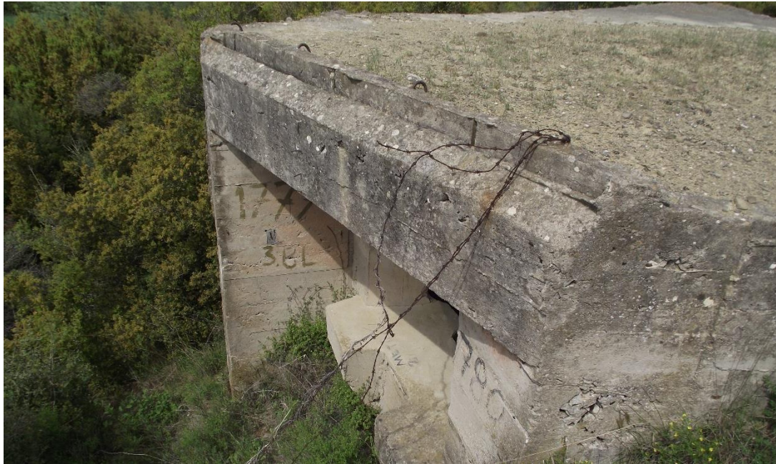
Figure 4.8 Bunker Type 1, front view photo with eaves and extension, Photographed by the author on 27/04/2019
