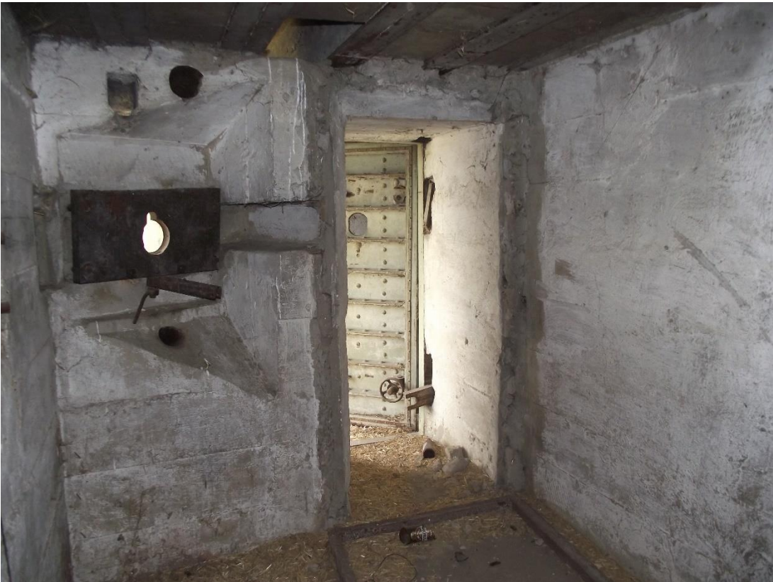
Figure 4.17 Bunker Type 4, hall and corridor, Photographed by the author on 25/04/2019
