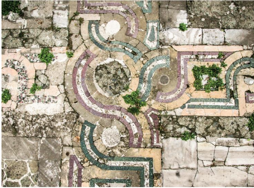
Figure 50: The Stoudios Monastery, opus sectile Floor Detail (Credit: © IBB KUDEB Arşivi, 2013)
