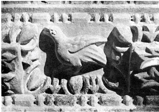
Figure 48: A Detail of Dentils on the Cornice of the Narthex Façade, 1929 (Credit: © German Archaeological Institute, Nicholas V. Artamonoff Collection)
