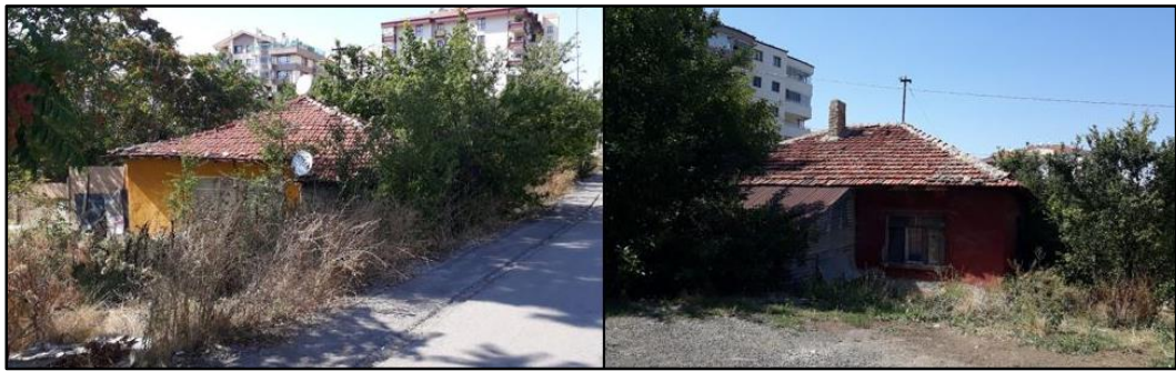
Figure 5.18. Neglected buildings - Çukurambar 33
