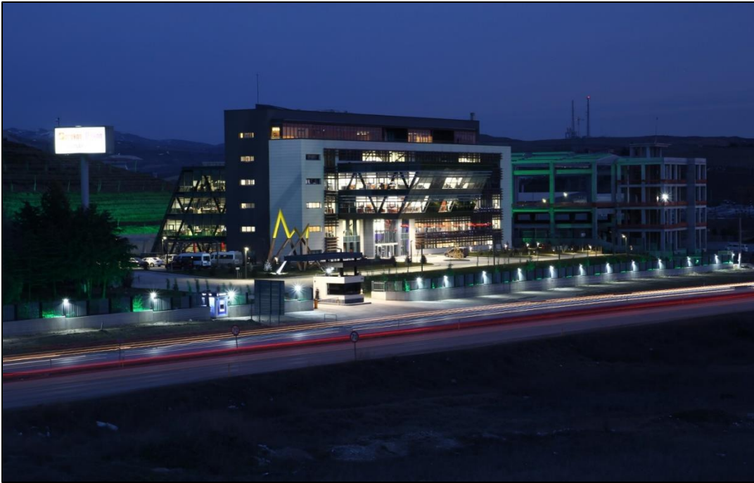
Figure 3.2. General view of Prokon-Ekon Office Building-II
