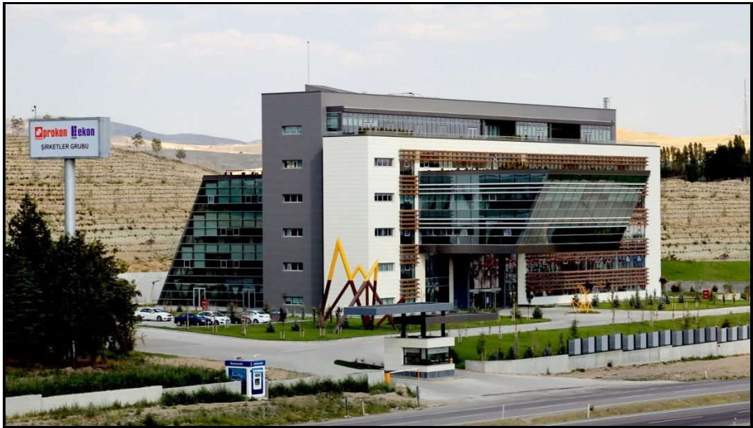
Figure 3.1. General view of Prokon-Ekon Office Building
