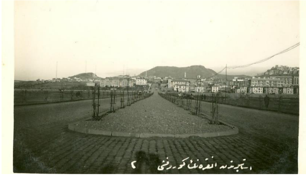
Figure 3.24: The view of Ankara for Station Square, with the buildings “gushed out” through the beautified İstasyon Caddesi , 1926-1927.
