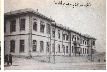
Figure 3.18.c: The new School of Industry and Mekteb-i Sanayi Avenue, 1900s.
