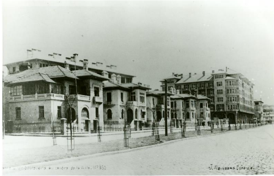
Figure 3.40: The view of Pious Houses and Blocks from İstanbul Avenue, 1930.
