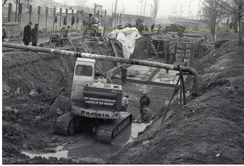
Figure.4.11. The construction work of closing İncesu Stream (Source: EskiAnkaraResimleri internet archive)
