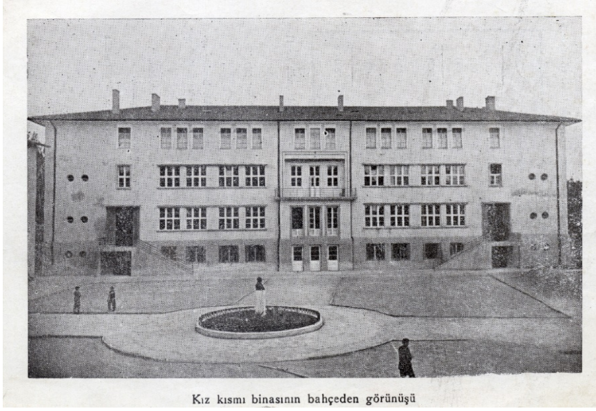
Figure.3.20. The back façade of G Block and a part of schoolyard (1955) (Source: TED Ankara College Private Schools archive)
