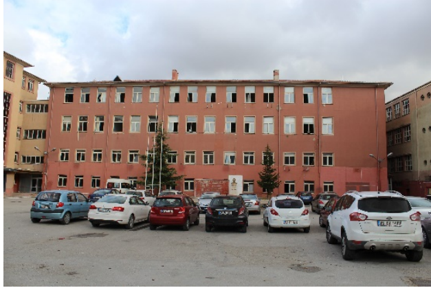
Figure.E.6. The A Block, 2013 (Source: Azize Elif Yabancı's personal archive)
