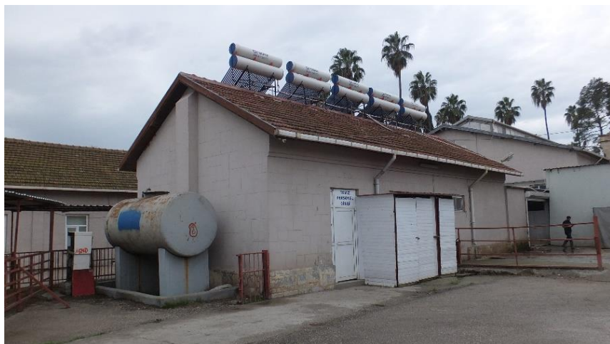
Figure 3.124. Exterior view of the dressing rooms
