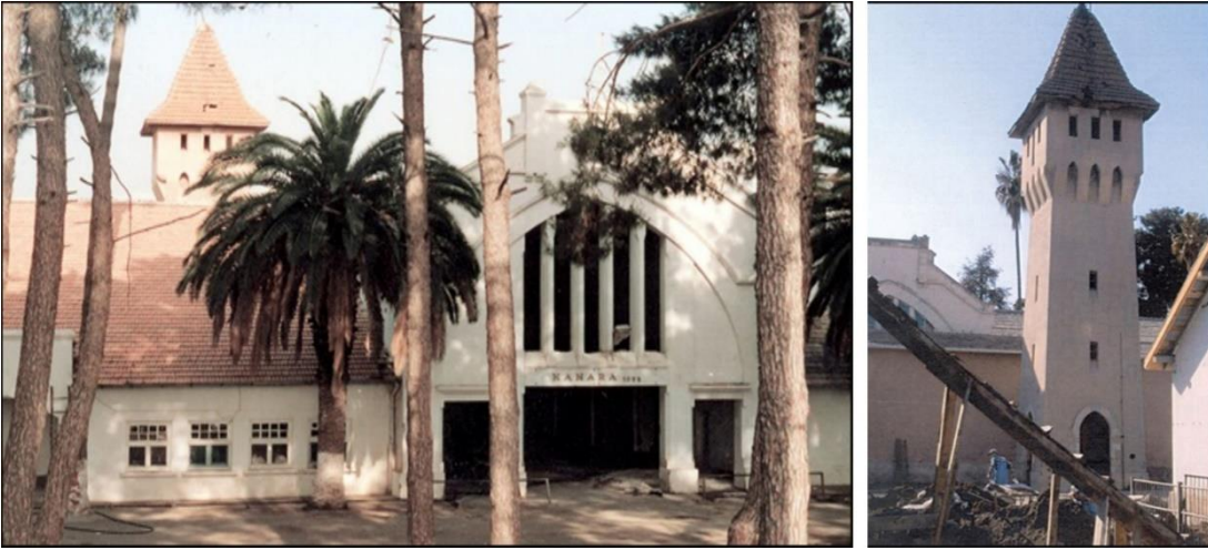
Figure 3.84. Kanara under repair after the abandonment (Source: Kültür Portalı retrieved from: https://kurumsal.turizm.gov.tr/turkiye/adana/kulturenvanteri/mezbaha--kanara )
