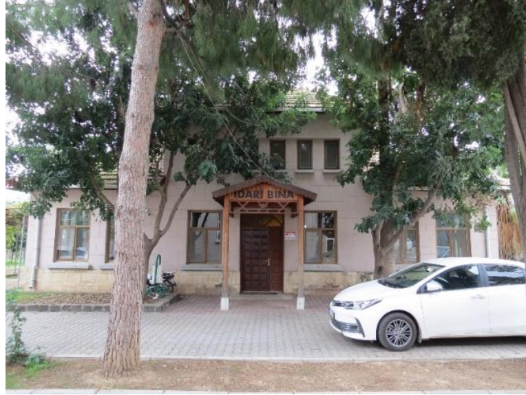
Figure 3.122. West façade of the administrative building
