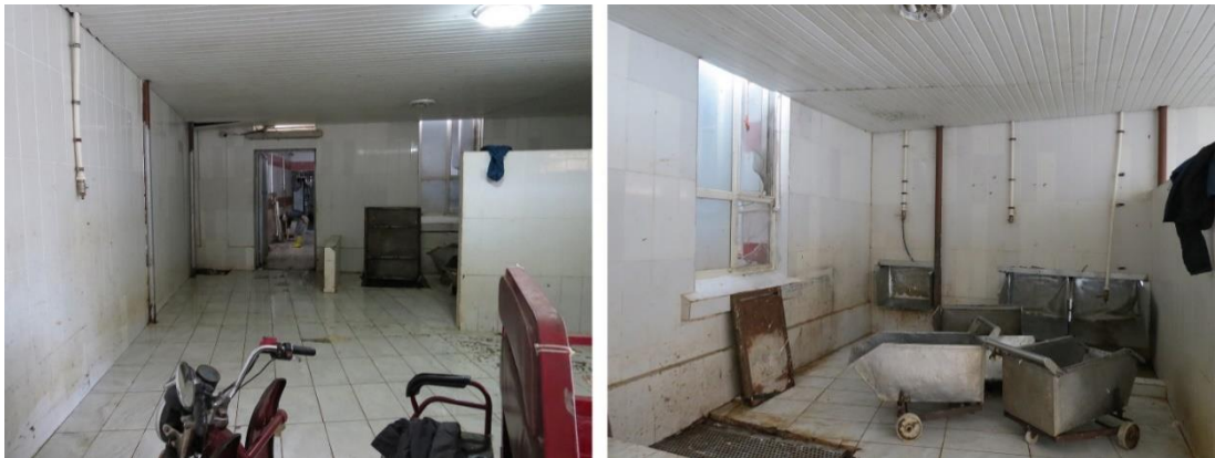
Figure 3.139. Interior view of the washing area
