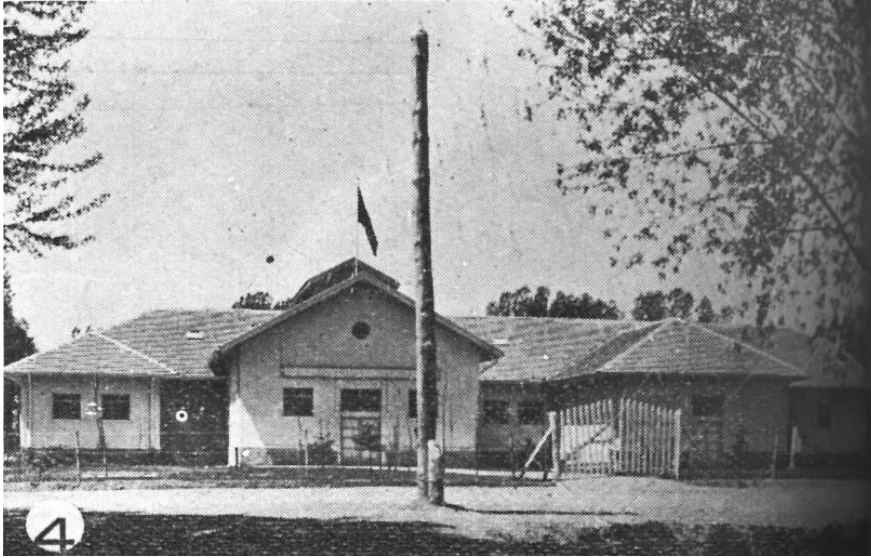
Figure 2.23. Sivas slaughterhouse (Source: İmamoglu, 2010, p.134)
