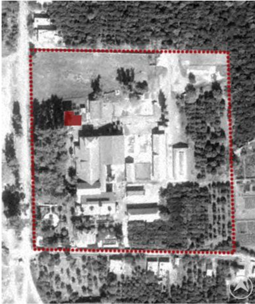
Figure 3.69. New transformer built between 1972 and 1985 (1985 Aerial Photo)
