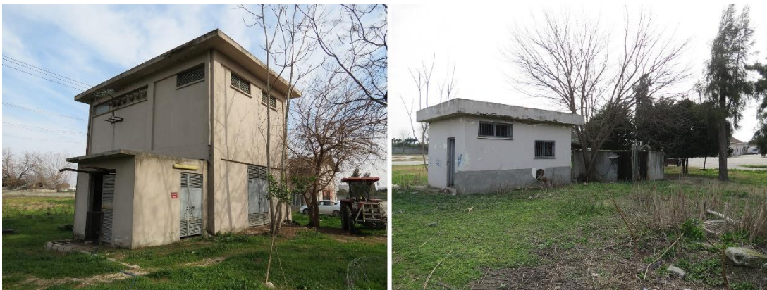
Figure 3.70. Transformer building (on left) and water pump building (on right)
