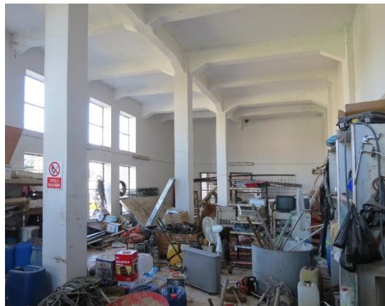
Figure 3.115. Interior view of the machine room
