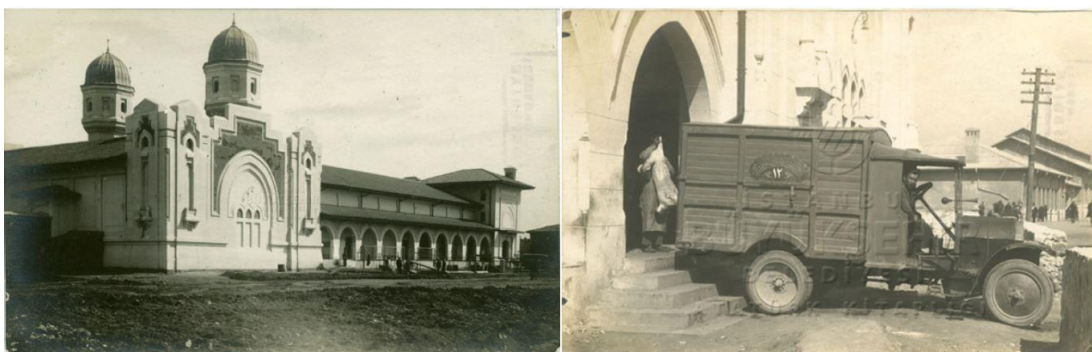
Figure 2.13. Cold storage building (Kucuk, 2015, p.243)
