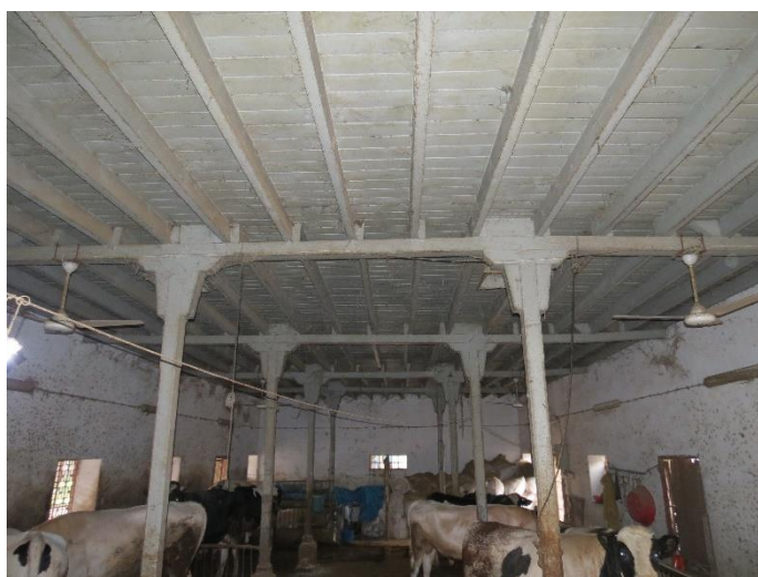
Figure 3.127. Interior view of the stable
