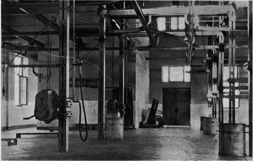
Figure 3.25. Interior view of the slaughter hall (Source: Temel, 1933, p.39)
