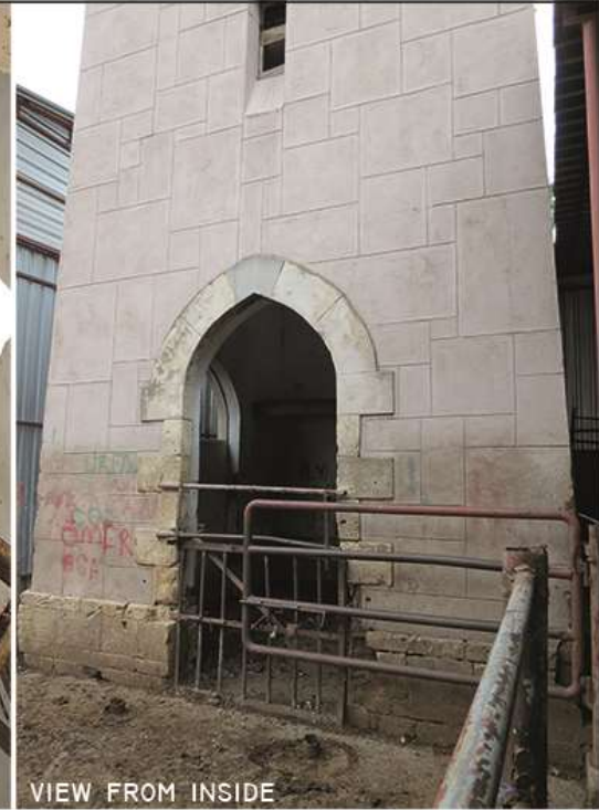
VIEW FROM INSIDE
