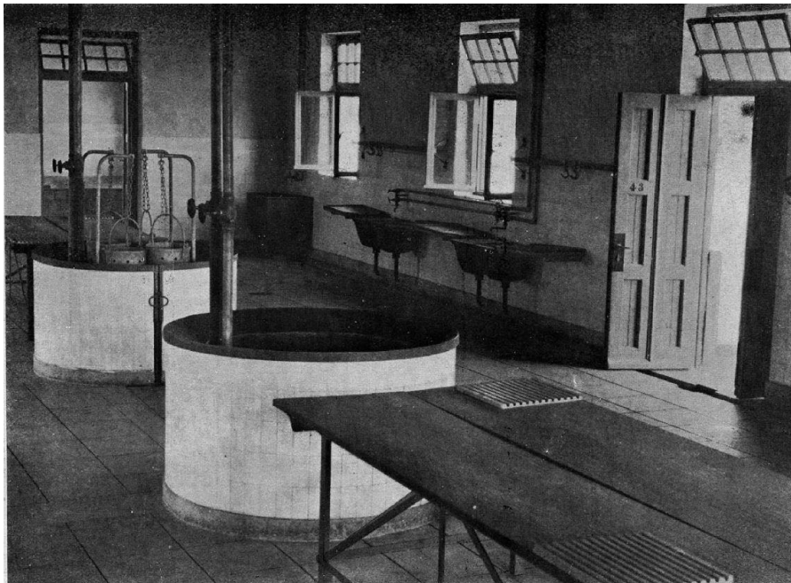
Figure 3.23. Interior view of cleaning tanks in paçahane (Source: Temel, 1933, p. 40)
