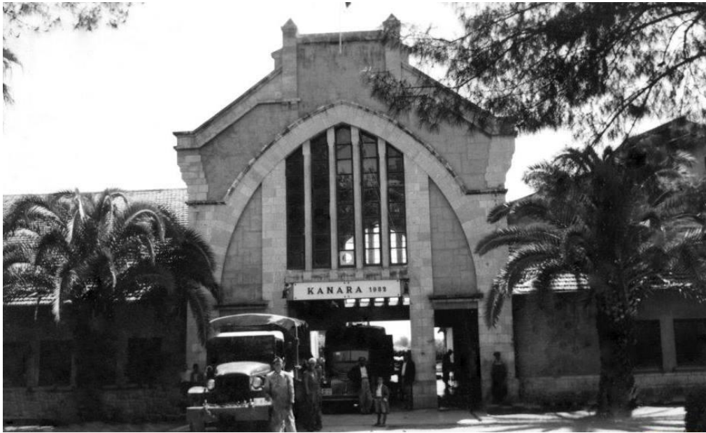
Figure 3.52. Trucks for transportation of meat in front of the slaughterhouse (Source: AEFEG)
