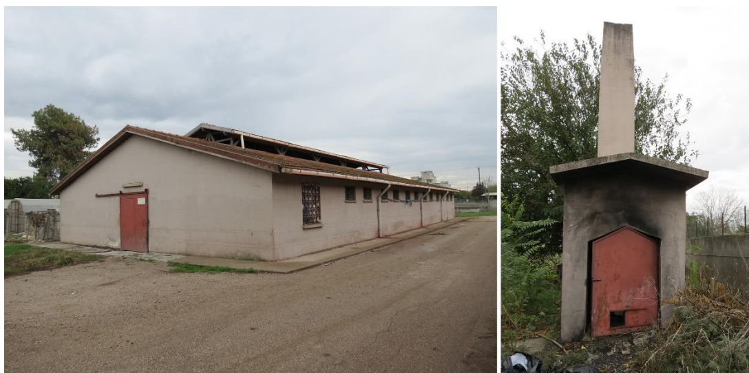
Figure 3.65. Second stable (on left) and annihilation room (on right)
