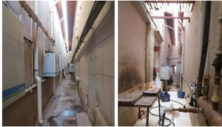
Figure 3.116. The space left between the slaughterhouse and cold storage depots
