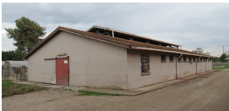
Figure 3.128. Exterior view of the second stable
