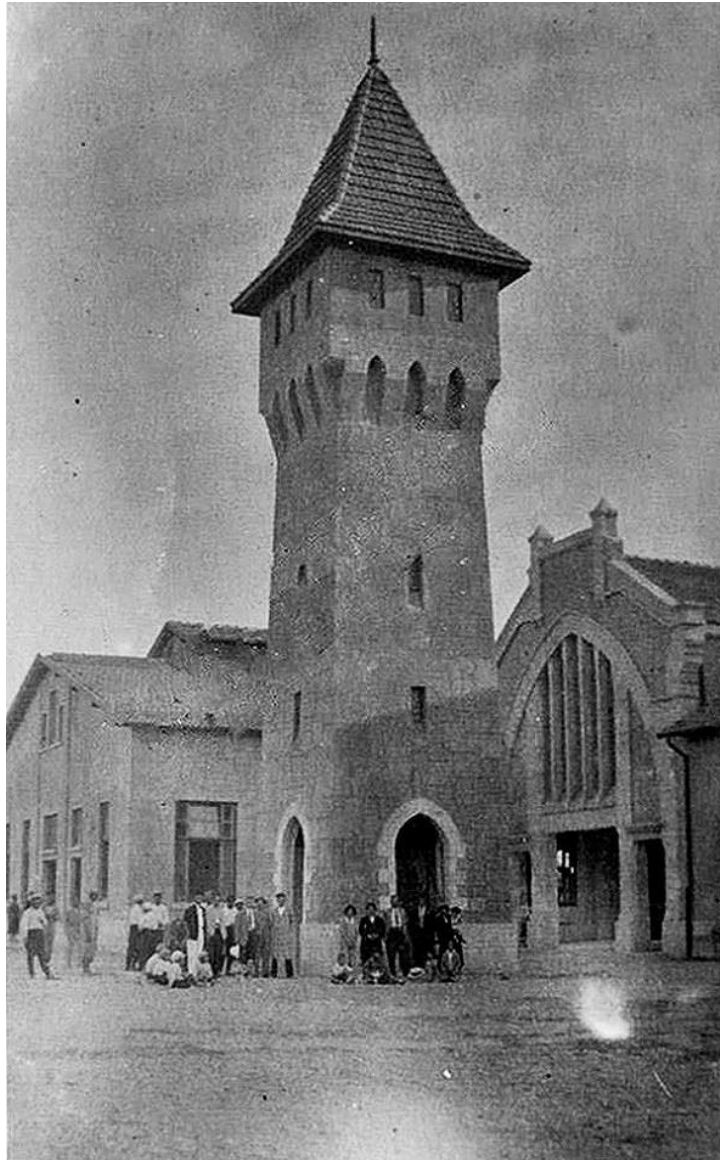
Figure 3.24. An old photograph of the water tower (Source: Adana Ansiklopedisi Facebook Group)
