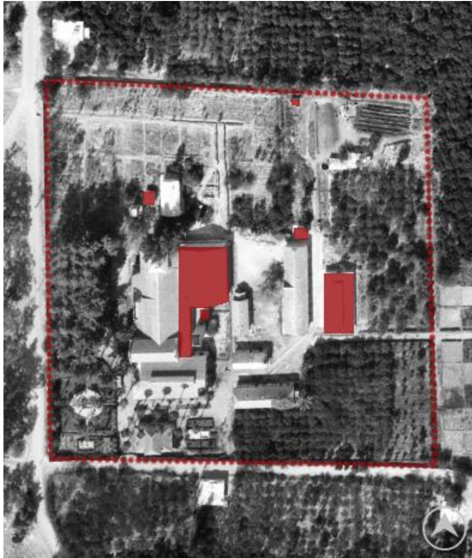
Figure 3.66. New buildings built in 1960s (1972 Aerial Photo)
