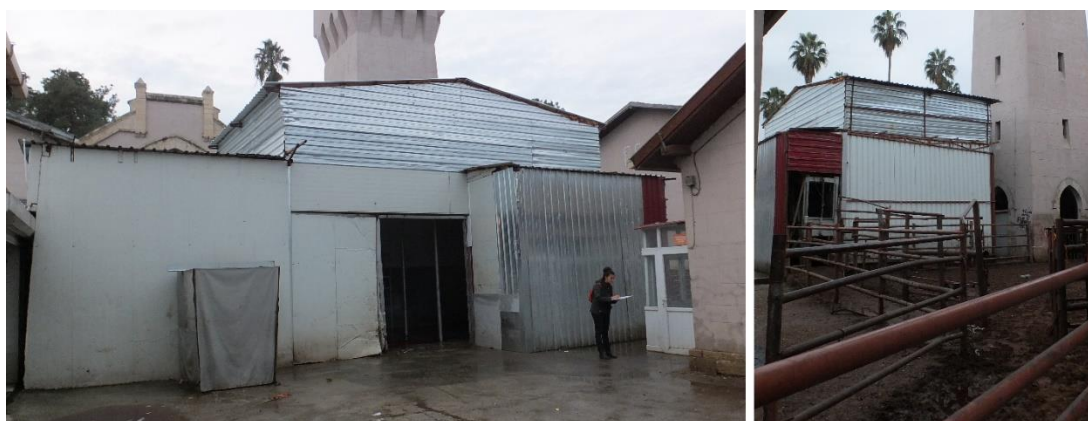
Figure 3.140. Exterior view of the new slaughter hall
