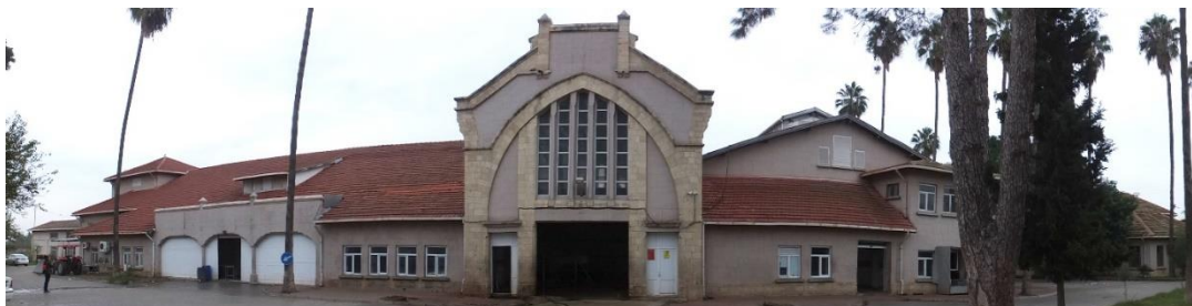
Figure 3.108. West façade of the slaughterhouse
