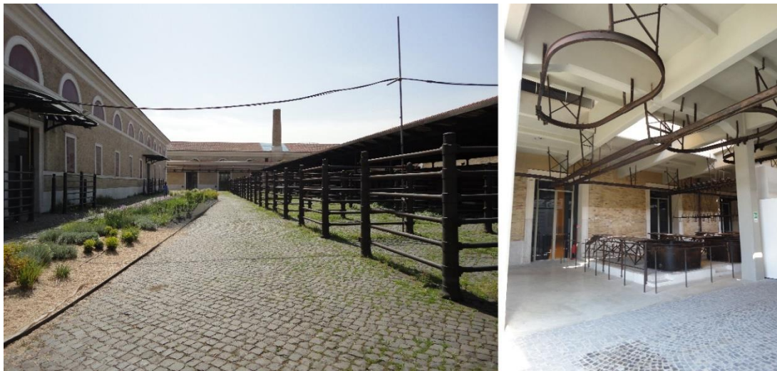
Figure 2.45. Exterior and interior views of the slaughterhouse, now used as an art center (Source: Güliz Bilgin Altınöz photo archive)
