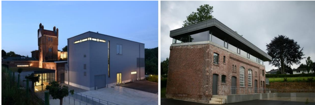
Figure 2.30. Additions and extensions of the former slaughterhouse complex (Source: http://www.dethier.be/en/projets/alter-schlachthof-cultural-center# )
