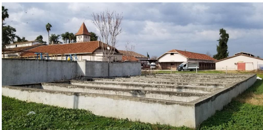
Figure 3.137. Water treatment pools
