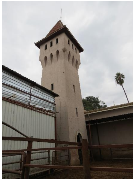
Figure 3.131. Exterior view of the water tower
