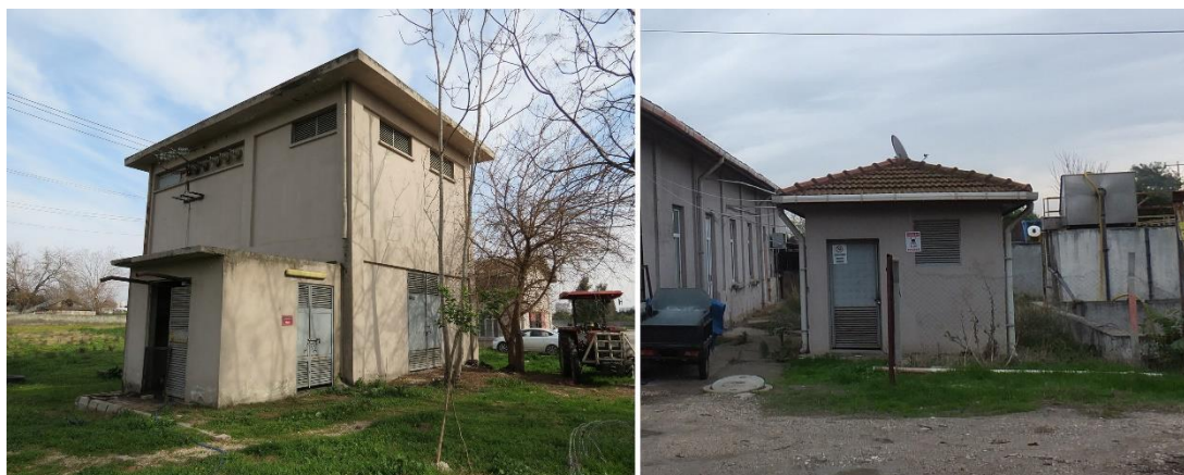
Figure 3.135. Transformer buildings (14) and (15)
