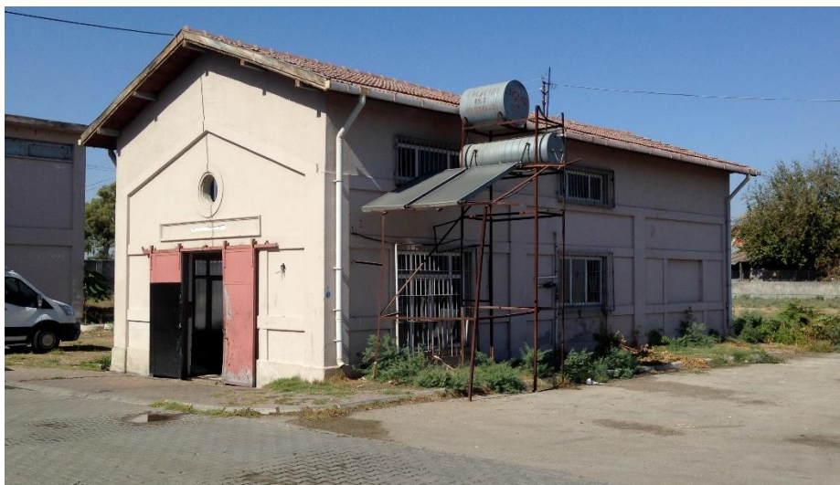
Figure 3.130. Exterior view of the bağırsakhane
