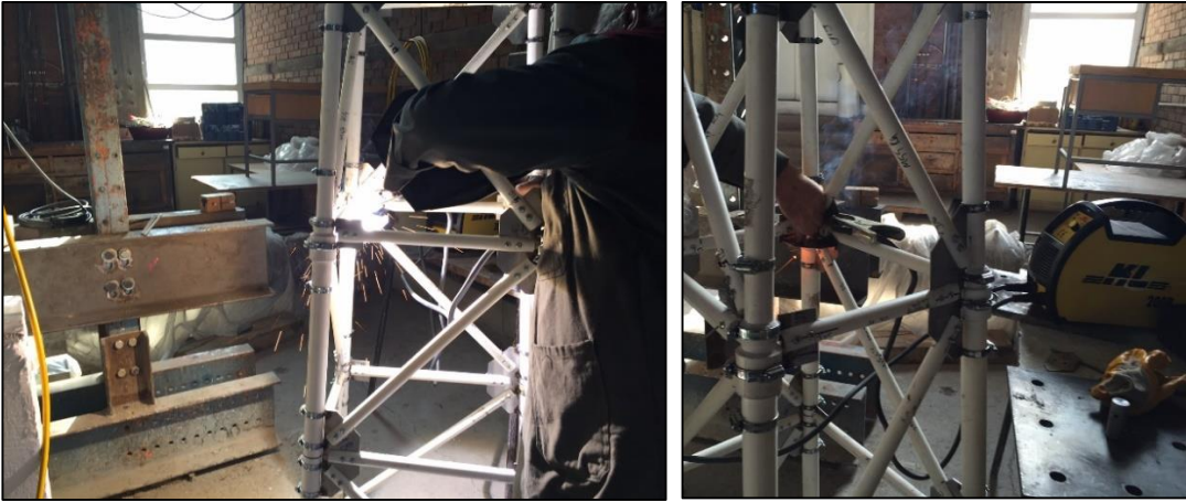
Figure 3.5. Welding Process of Connection Plates
