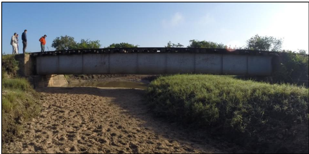
Figure 4.6. The upstream side of the existing bridge (Cur_BR01)
