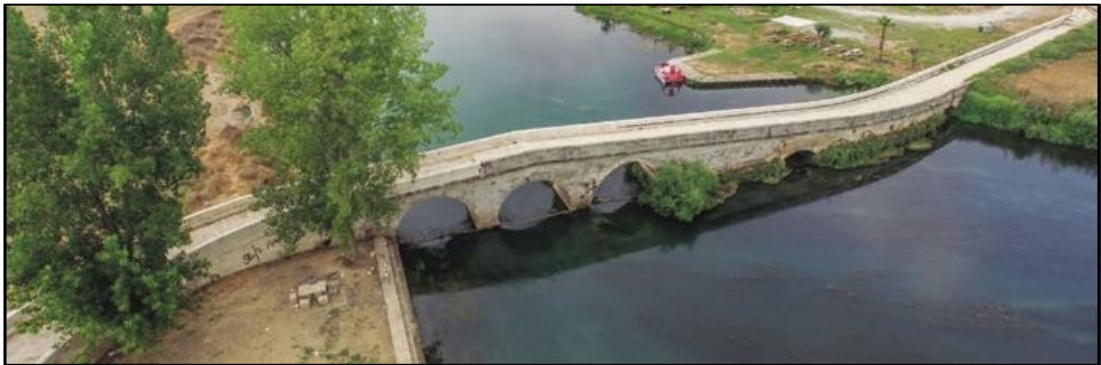
Figure 5.1. The current state of the Düden (Cırnık) Bridge (upstream side)
