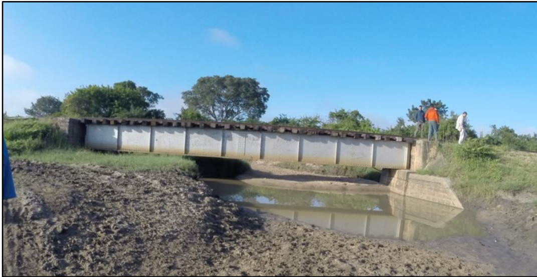
Figure 4.7. The downstream side of the existing bridge “Cur_BR01”
