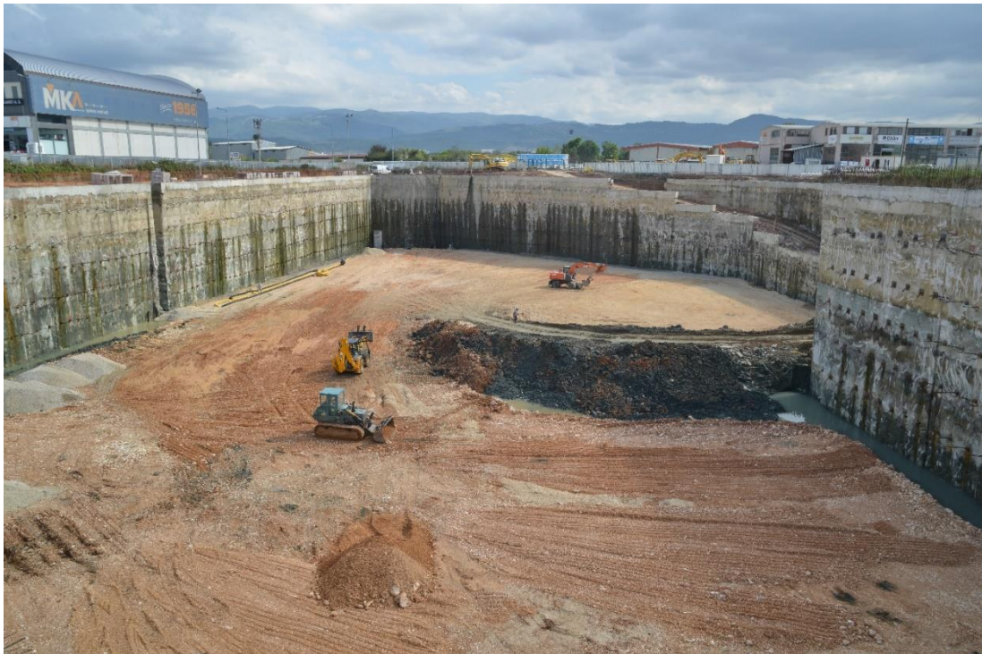
Figure 1.1. Özdilek Shopping Mall (24 m of Diaphragm Wall) – Bursa, Turkey – The Fourth Highest Population in Turkey with 2.9 Million
