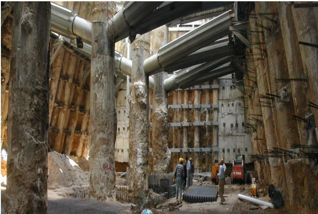
Figure 1.2. Ankara Metro 3. Stage Kızılay Retaining System (35 m Deep Station) – Ankara, Turkey – The Second Highest Population in Turkey with 5.5 Million
