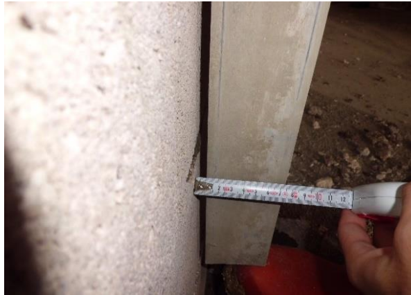
Figure 4.5 Photos from site inspections
