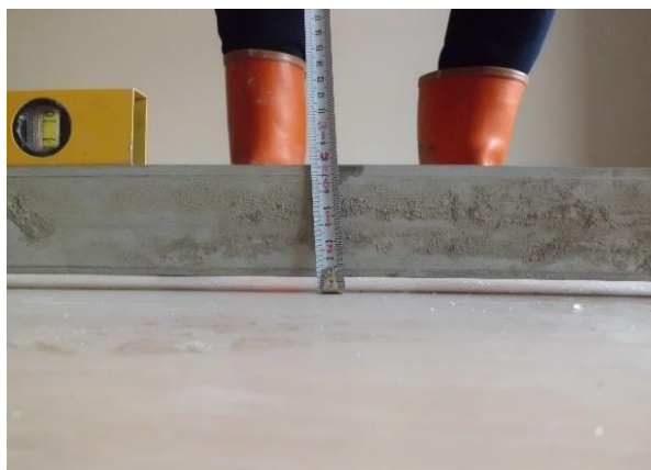
Figure 4.6 Photos from site inspections
