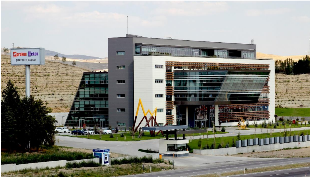
Figure 3.1. Picture of Prokon Ekon Headquarter Building
