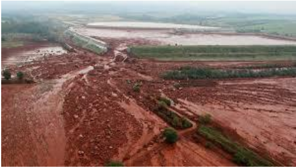
Figure 2-4. Collapsed red mud dam in Hungary (Gyoergy Varga /AP)
