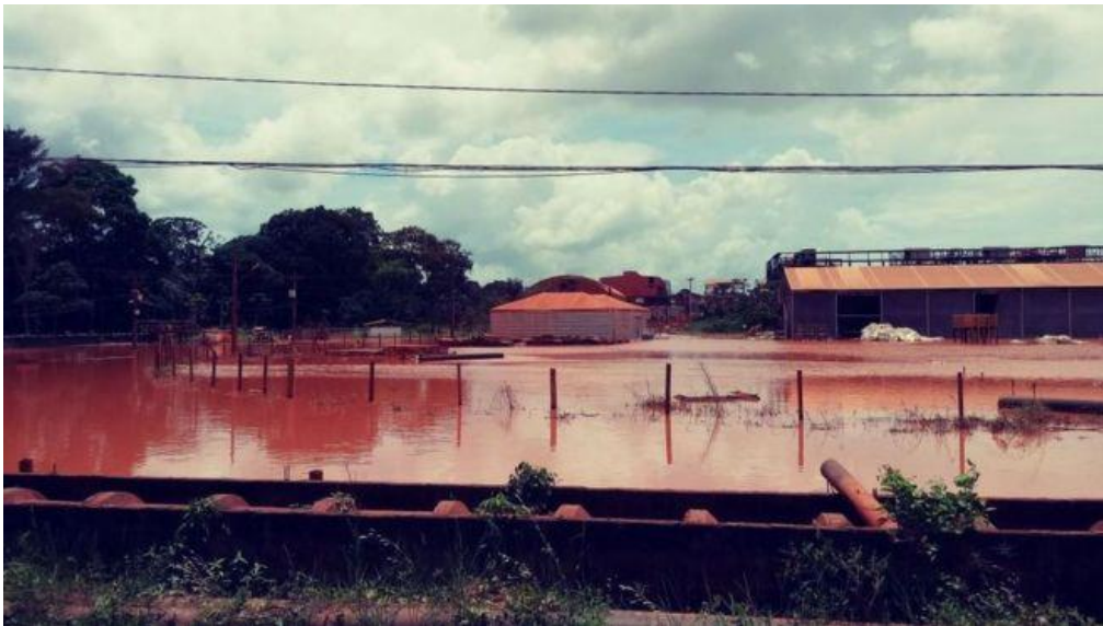
Figure 2-3. Spilled red mud dam in Brazil (Instituto Evandro Chagas, 2018)
