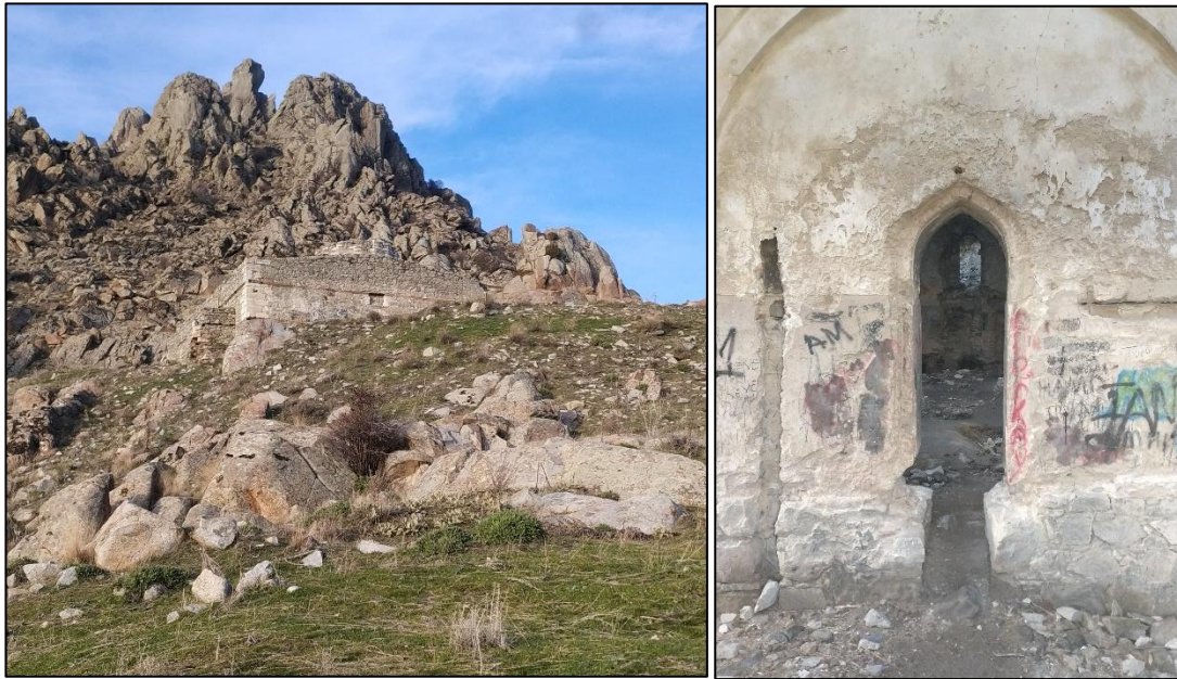
Figure 4-64. Gavur Hamamı (the Armenian Bath) from the Outside (left) (Author, March, 2019) and Inside of the Bath (right) (Author, March, 2019)
