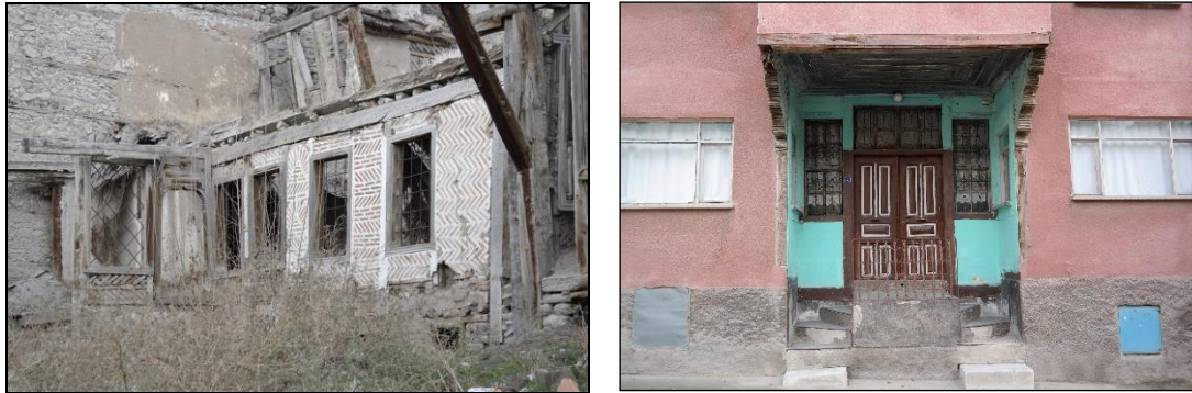
Figure 3-36. Decorative Figures on Walls (Left), Ornaments on Façade Elements (Right) (Author, December, 2017)
