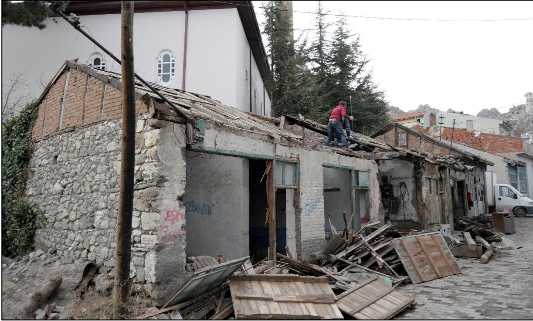
Figure 4-7. The Demolition of the Shops around Aziz Mahmud Hüdai Mosque (Author, December, 2017)
