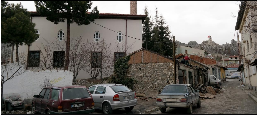
Figure 4-32. Demolition of the Shops in Demirciler Arastası (Author, December, 2017)
