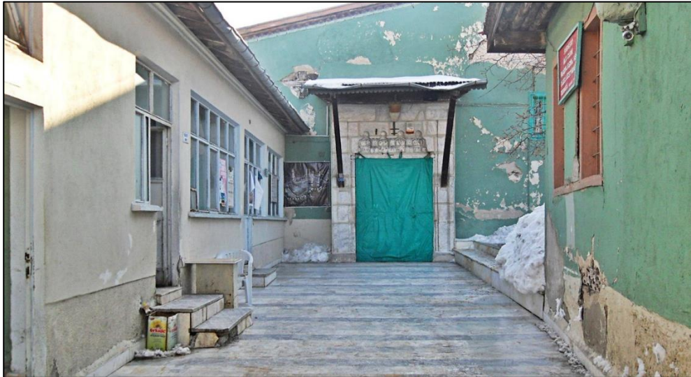
Figure 4-46. The Entrance of the Great Mosque before Restoration (Şenol Öz's Personal Archive)
