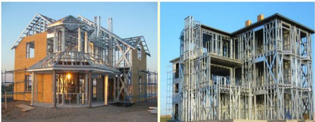
Figure 1.1 CFS structural systems
