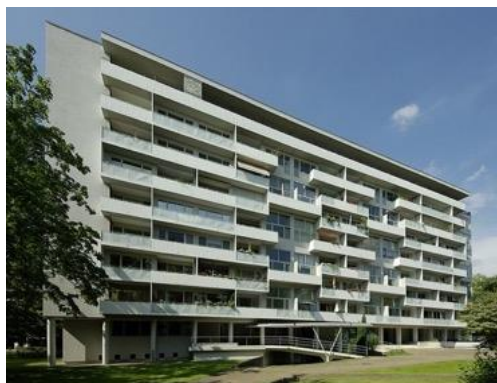
Figure 4.51. Building no.21 view Source: https://www.archinform.net/projekte/11820.htm
