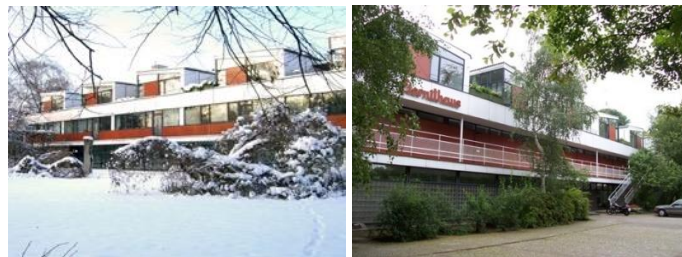
Figure 4.62. Building no.25 south façade
