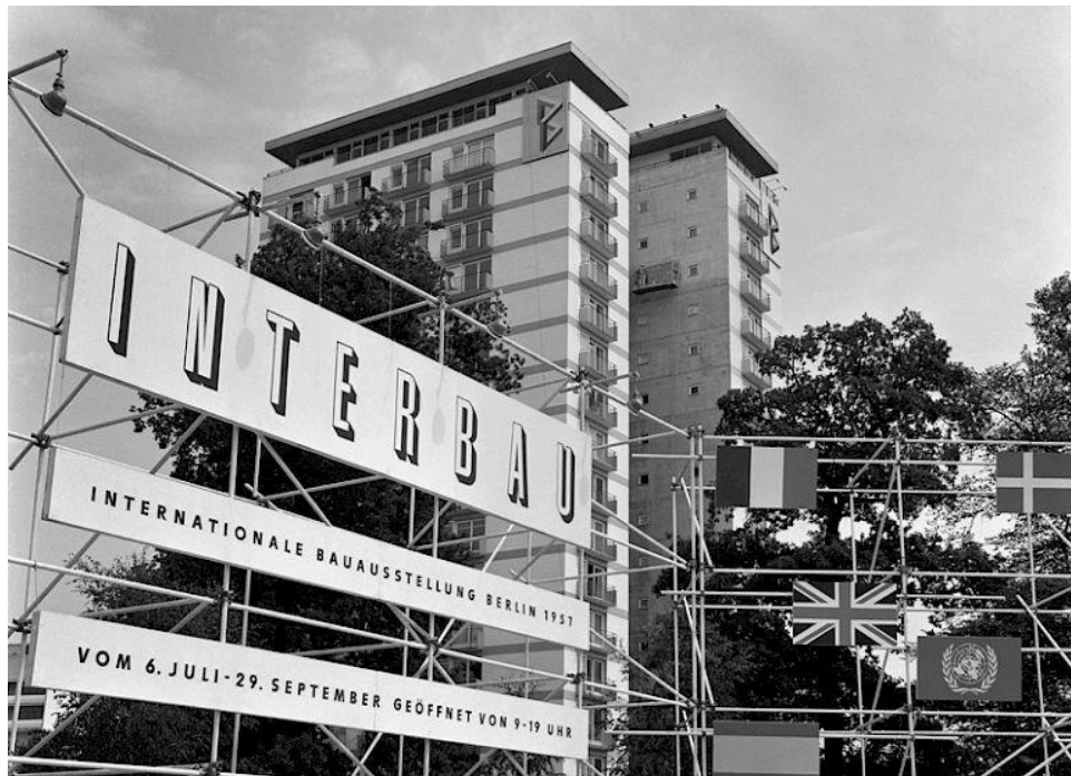
Figure 2.1. Entrance to the Interbau in the Hansaviertel District, 1957 Source: © Landesarchiv Berlin, F Rep. 290 Nr. 0054972 / Image: Willy Kiel
