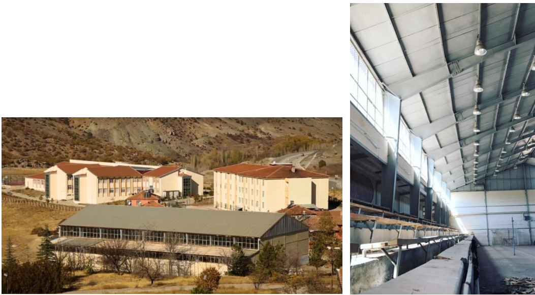
Figure 4-22. Sports saloon Source: Chamber of Architects Ankara Branch archive (2017)
