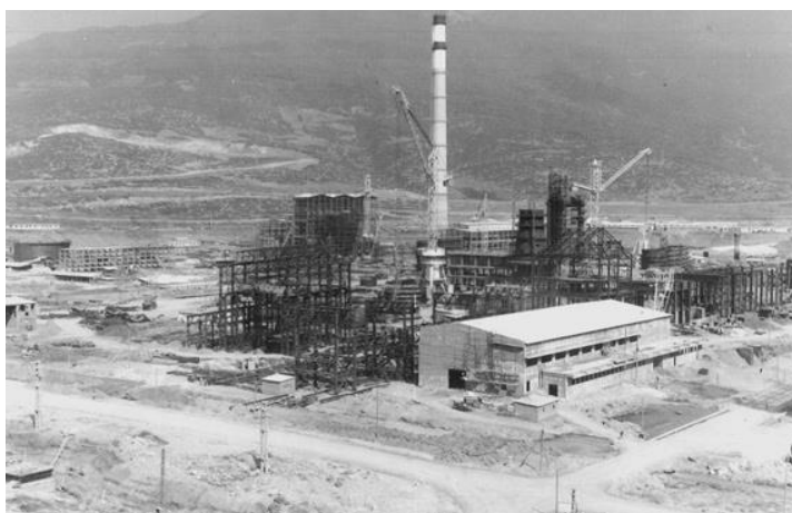
Figure 3-4. Start of the first stage of İskenderun Iron-Steel Factories in 1972
