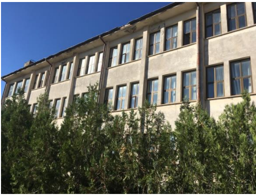
Figure 5-19. Administrative building Source: Taken by author
