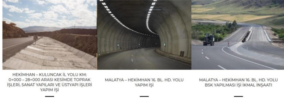
Figure 5-9. Images from the road and tunnel projects
