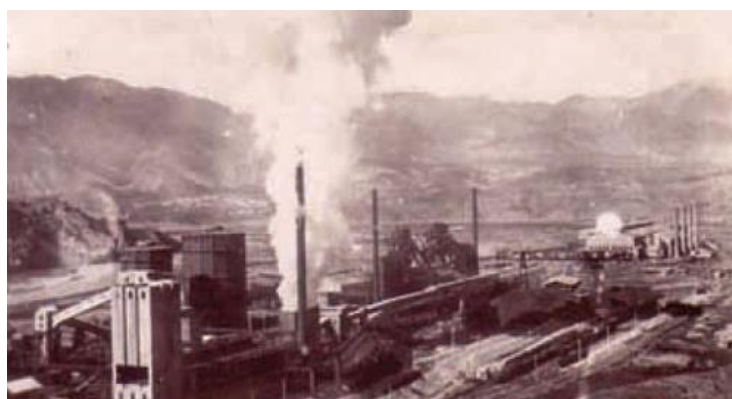
Figure 3-1. Karabük Iron and Steel Factory in 1937
