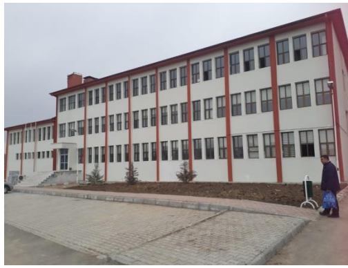
Figure 5-20. Hekimhan Municipality building Source: Firat, C. (2019), Taken by municipality staff
