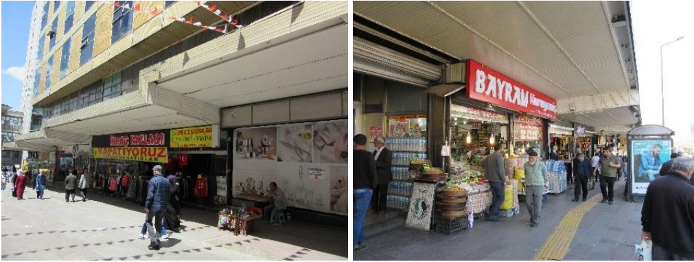
Figure 3.23. The wide eaves on the longer facades (Author, 2019)
