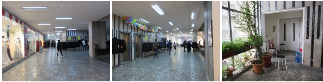
Figure 3.36. Photos of mezzanine in E block (Author, 2019)
