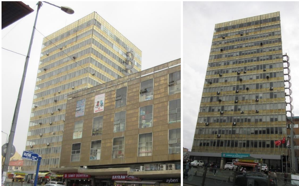
Figure 3.27. The Anafartalar Street Facade of high-rise office block (Author, 2017)
