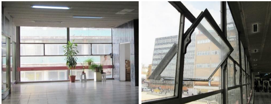
Figure 3.49. The window arrangement on the curtain walls and the horizontal pivoting window (Author, 2019)
