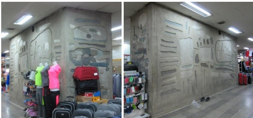
Figure 3.64. The sgraffito mural painting of Adnan Turani in the 3rd floor (Author, 2017)
