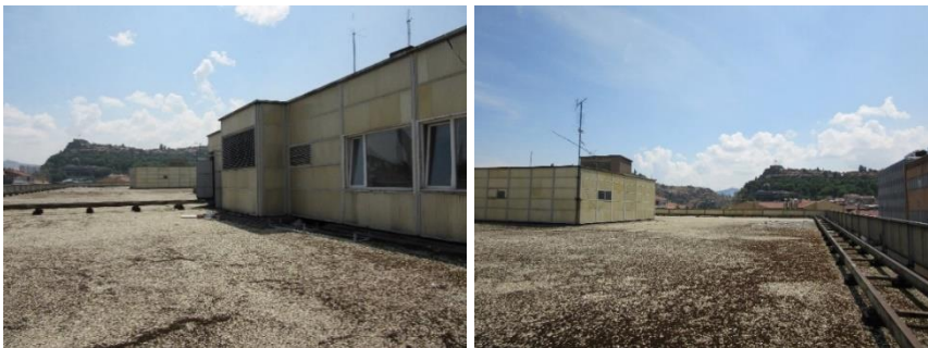
Figure 3.40. The two low-rise masses on the flat roof (Author, 2019)
