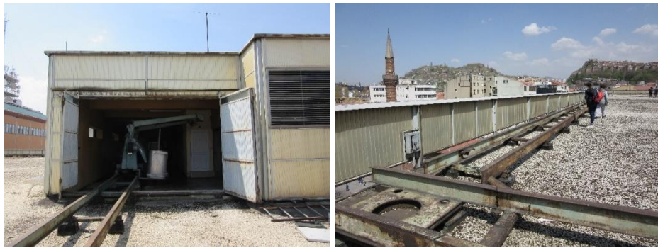
Figure 3.48. The façade elevator and its mechanism with rail (Author, 2019)
