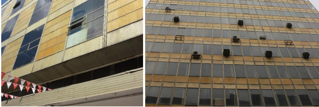
Figure 3.28. The hue changes in the aluminum modules: in Anafartalar Çarşısı (left), in high-rise block (right) (Author, 2017)
