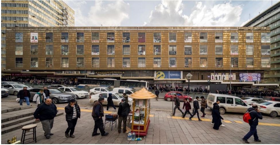
Figure 3.24. The North Elevation: The Anafartalar Street façade (Source: Galip Kürkcü Archive)
