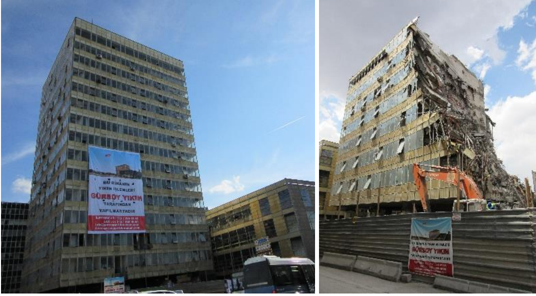
Figure 3.74. Photos from the demolition of the office block (Author, 2018)
