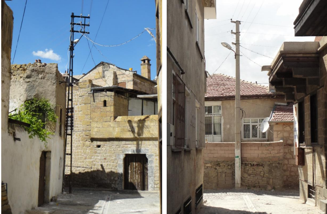
Figure 3.71. Lights on utility poles (Personal Archive)
