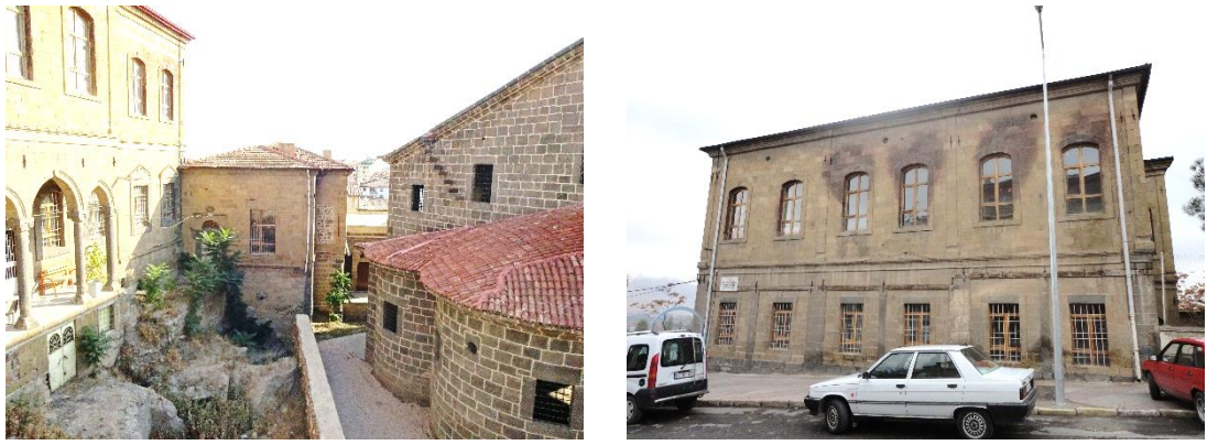
Figure 3.57. Dumlupınar Primary School (Personal Archive)
