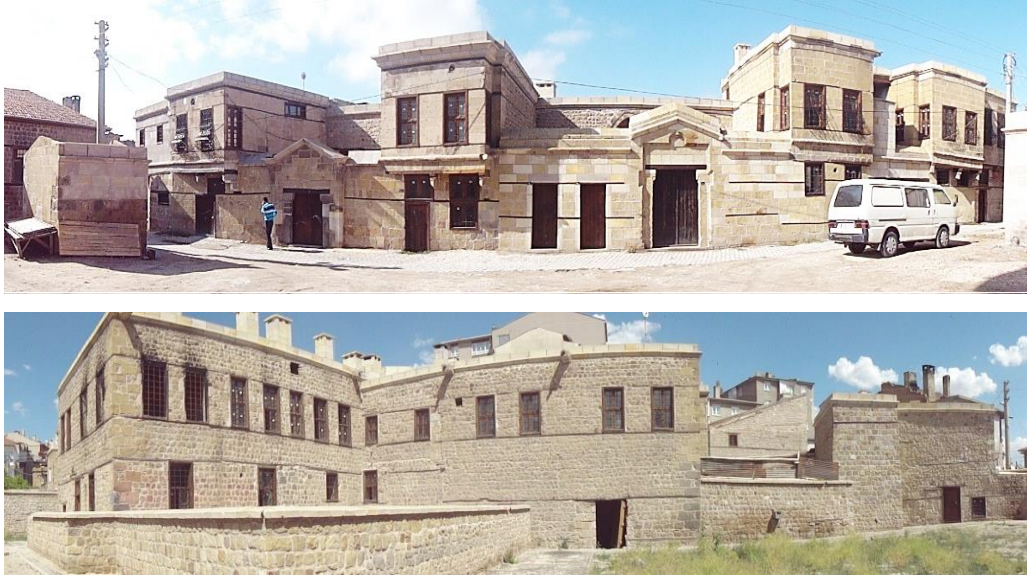
Figure 2.30. Traditional residential buildings that are repaired within the scope of the CSRP (Personal Archive)
