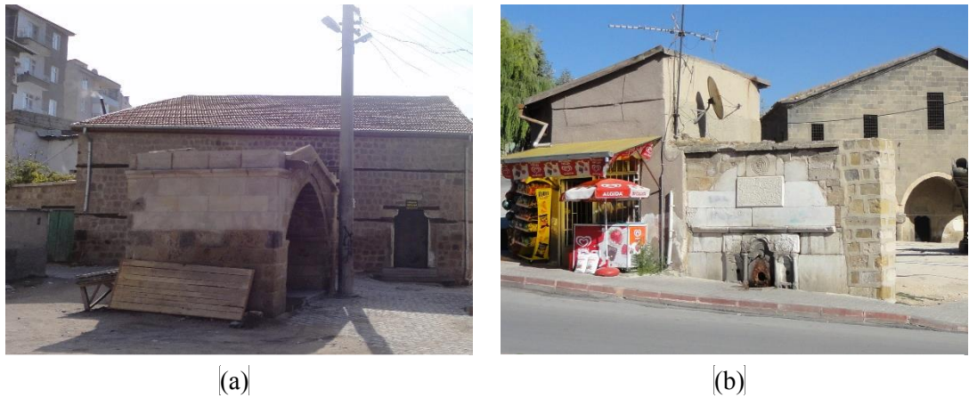
Figure 3.53. (a) Cullaz Masjid and Fountain (b) Nalbantlar Fountain (Personal Archive)
