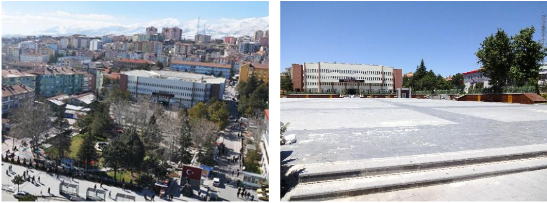
Figure 3.5. Before and after photographs of the city square ( http://nigde.bel.tr , Personal Archive)
