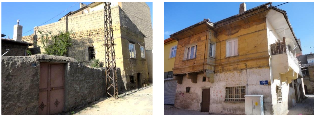
Figure 3.43. Changes in traditional houses (Personal Archive)
