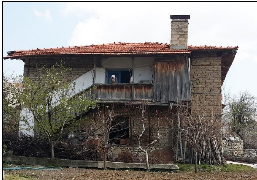
Figure 94: Southwest facade of the H15. An example for the chimney and the eave, extending over the 'gezenek' on which the toilet is located.
