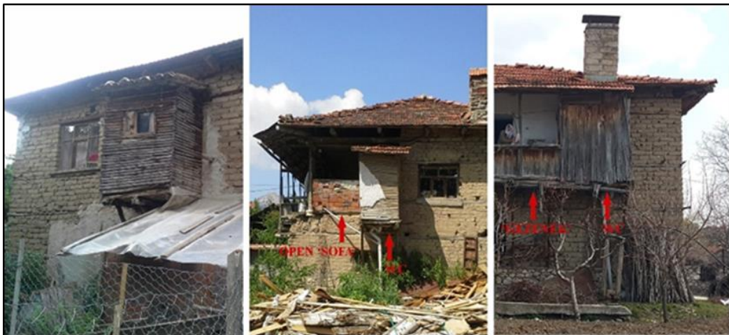
Figure 132: First photo shows the toilet located at the end of the 'enlarged corridor'(H11); the second one shows the toilet located adjacent to the open 'sofa'(H16); the last one shows the toilet located at the end of the 'gezenek'(H15).
