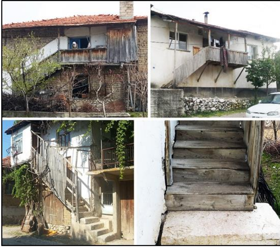
Figure 63: The photos from the H11, H15 and H19; wooden staircases which reach the 'gezenek', the 'balcony' and the 'sofa' on the first floors.
