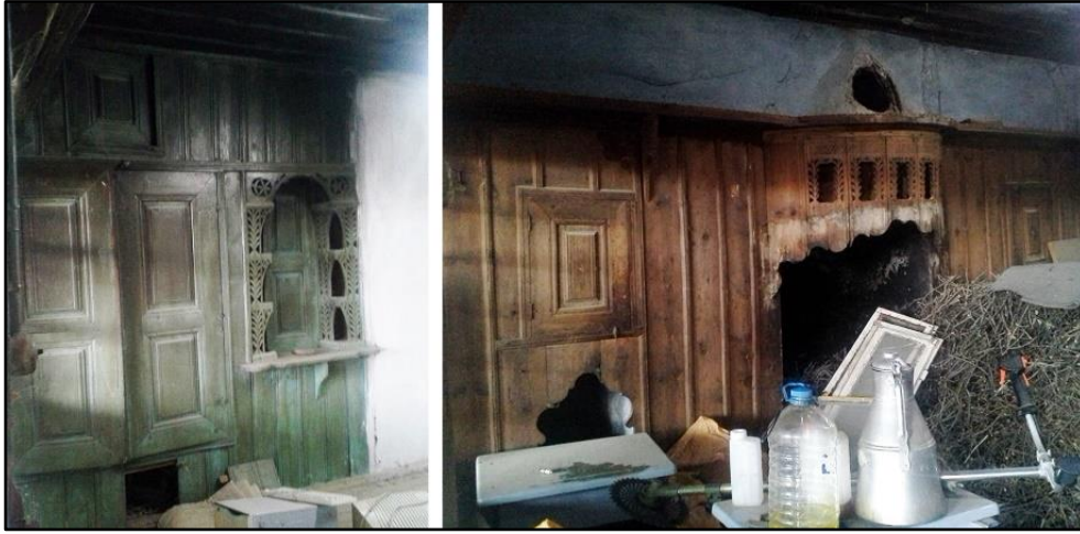
Figure 147: A 'Yüklük', a 'şerbetlik' and an 'ocak' with a 'yaşmak'. The photos are from the H13.
