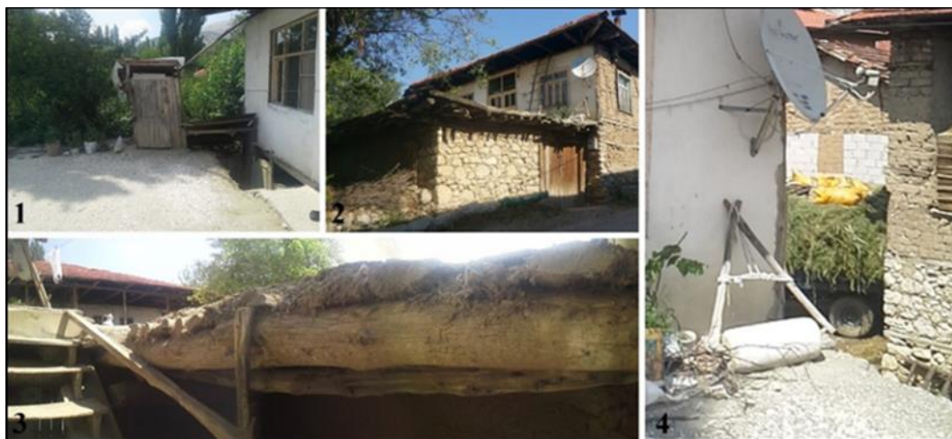
Figure 55: The first photo shows the surface of the original ‘saçak’; the second one shows the relation between the ‘saçak’ and the main mass of the house; the third one shows the layers of the ‘saçak’ structure; the fourth one shows the ‘yuvga’ stone. All photos are from the H4.
