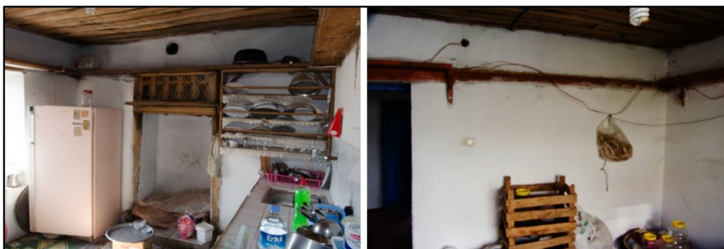
Figure 70: Tereks on the walls of the H15. The photo on the left is from the space used as a kitchen while the photo on the right is from one of the rooms.
