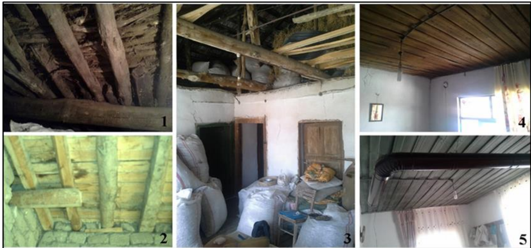
Figure 92: The first photo, showing the relation between ‘ döver ’, ‘ mertek ’ and ‘ pargi ’, is from the ground floor of the H14; The second photo, showing the relation between ‘ döver ’, ‘ mertek ’ and floor boards, is from the ground floor of the H15; the third one shows the ‘ sofa ’ without ceiling covering; the last two photos shows the same type of ceiling with different colours belonging to the rooms of H5 and H4 respectively.
