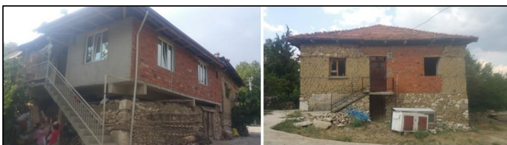
Figure 20: The structural transformation of the traditional mud brick masonry houses in Ağlasun.
