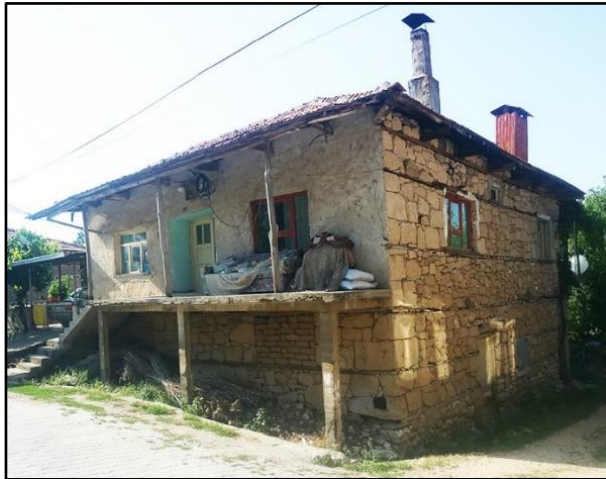
Figure 18: The traditional house, completely built with stone masonry construction technique.
