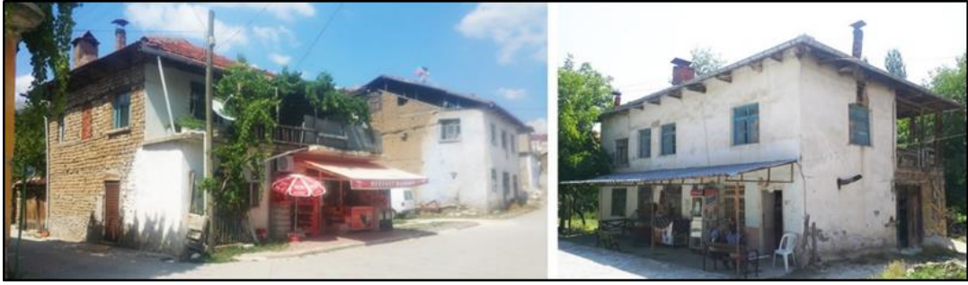
Figure 9: Photos on the both left and right sides show that two storey traditional mud brick masonry houses whose ground floors are used as grocery shops of neighbourhoods that they exist.
