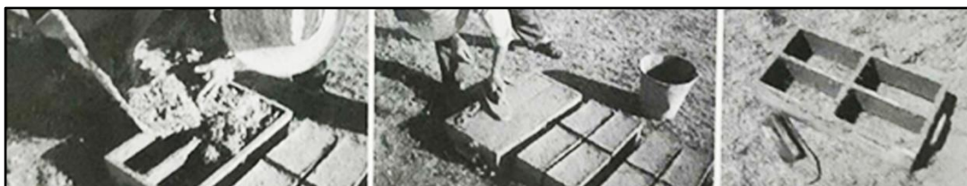
Figure 30: Mud brick production with traditional molds and equipment. (Cookson, 2010, as cited in Kafescioğlu, 2017, p. 106)
