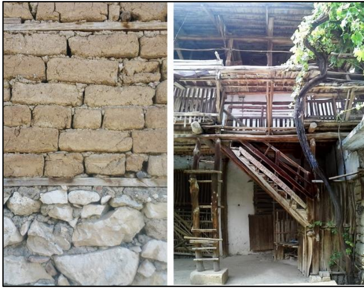
Figure 145 : Stone, mud brick and timber, the local construction materials of the Traditional Houses in Ağlasun. The photo on the left is from the H15 and the photo on the right is from the H9.
