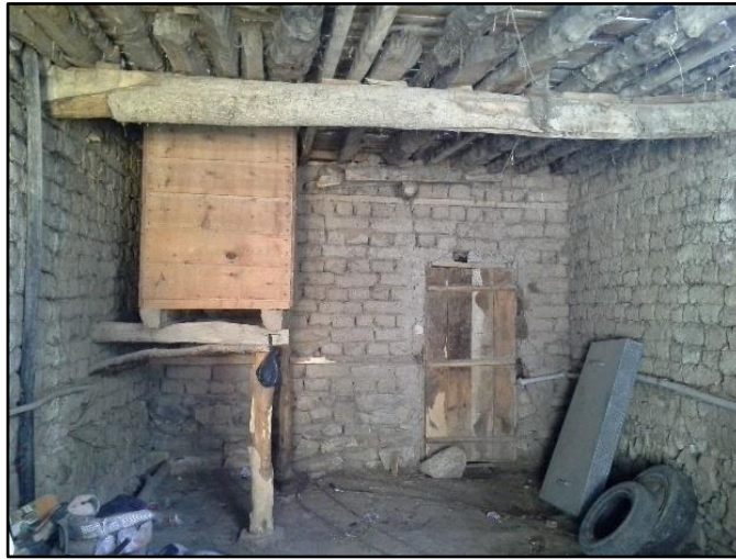
Figure 42 : The granary located on the wooden pillars with stone bases in the ground floor of a main building.
