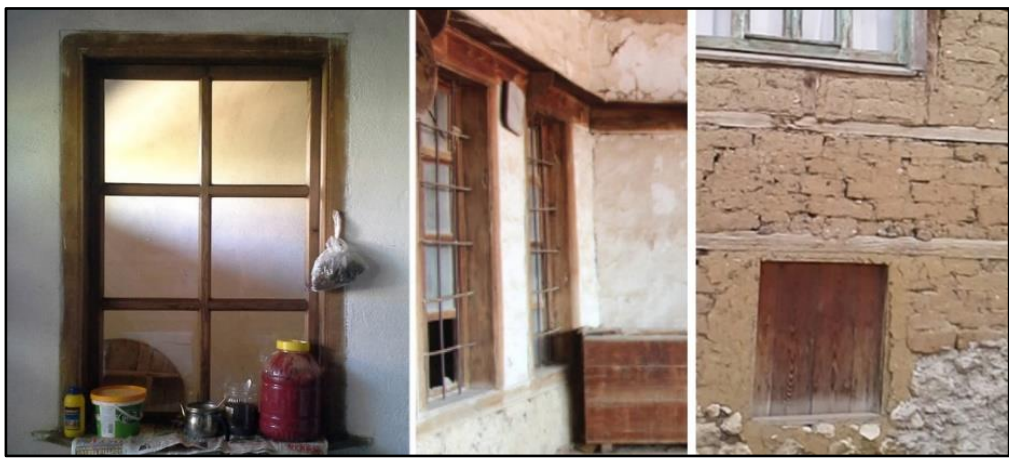
Figure 68: On the left, the window between the room and the closed ‘sofa’ in the H1; the image, produced by utilizing the study ‘Understanding a Historic Rural Landscape in Relation with an Archaeological Site: Ağlasun/ Sagalassos’, shows the windows between the room and the open ‘sofa’; the photo from the H4, shows the opening called ‘samanlık’.
