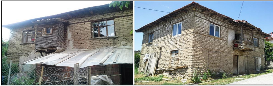
Figure 76: The photo on the left from the H11, shows the toilet located on the facade facing to the garden and the photo on the right from the H15 shows the balcony on the facade facing to the street.
