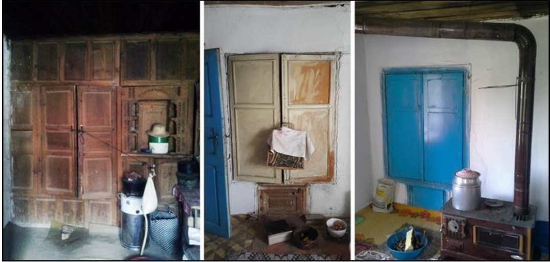
Figure 71: On the left, the ‘yüklük’ in the H7 which serves to just one room; on the right, the ‘yüklük’ in H15 which serves to the rooms located both side of it.
