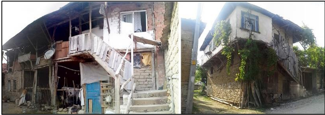
Figure 75: The photo on the left from the H13, shows the two storey main building with the open 'sofa' and the staircase on its courtyard facade; the photo on the right from the H19, shows the main building with mezzanine and the closed 'sofa' constructed as a projection.
