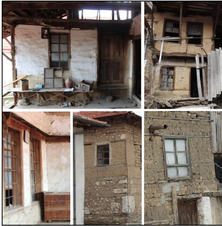
Figure 101: Window types of Traditional Mud Brick Masonry Houses in Ağlasun. Image is produced by utilizing photos from ‘Understanding a Historic Rural Landscape in Relation with an Archaeological Site: Ağlasun/ Sagalassos’ 15
