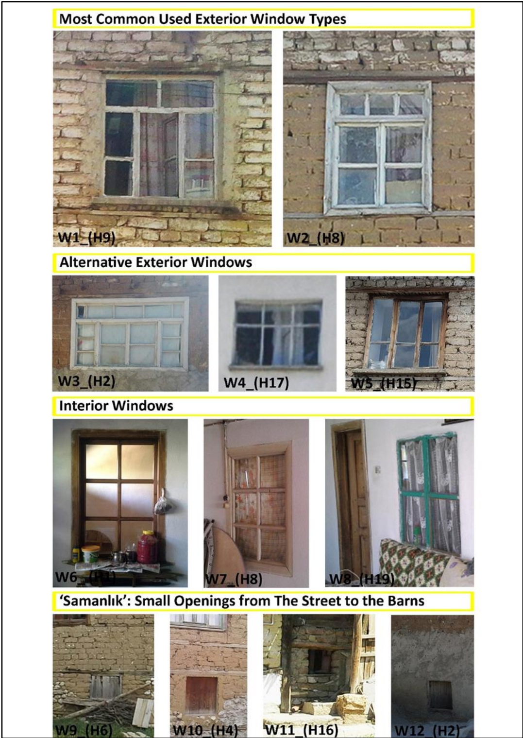
Figure 100: Window types of Traditional Mud Brick Masonry Houses in Ağlasun.
