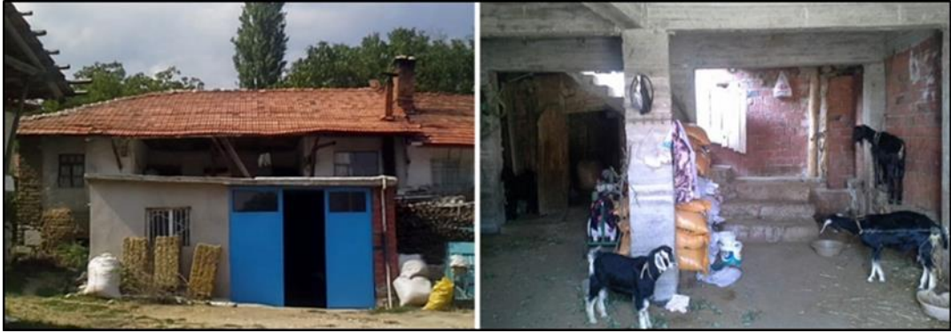
Figure 56: Two photos from the H5 show the 'saçak' that is constructed with reinforced concrete and the circulation area built with hollow bricks beneath the 'saçak' structure. The photo on the left shows the window and door of it and the one on the right shows the circulation space located under the 'saçak' structure.
