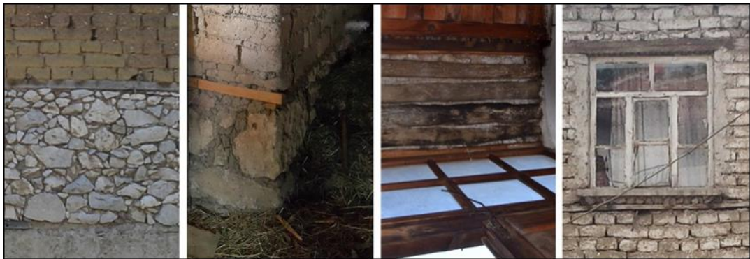
Figure 79: From the left to the right: rubble stone masonry (H3); cut stones at the corners of the stone masonry part of the wall (H15); ‘helik’ stone as infill material over a door opening (H7); ‘helik’ stone usage as infill material under a window opening (H9).
