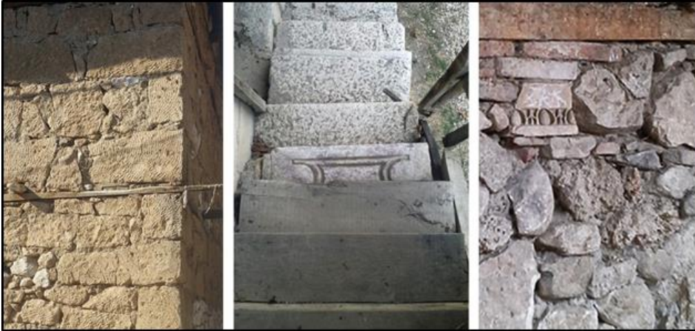
Figure 80: From the left to the right: the stone masonry with 'Köğke' stone; use of spolia as a step of the staircase (H19); use of spolia as a part of stone masonry wall (H13).
