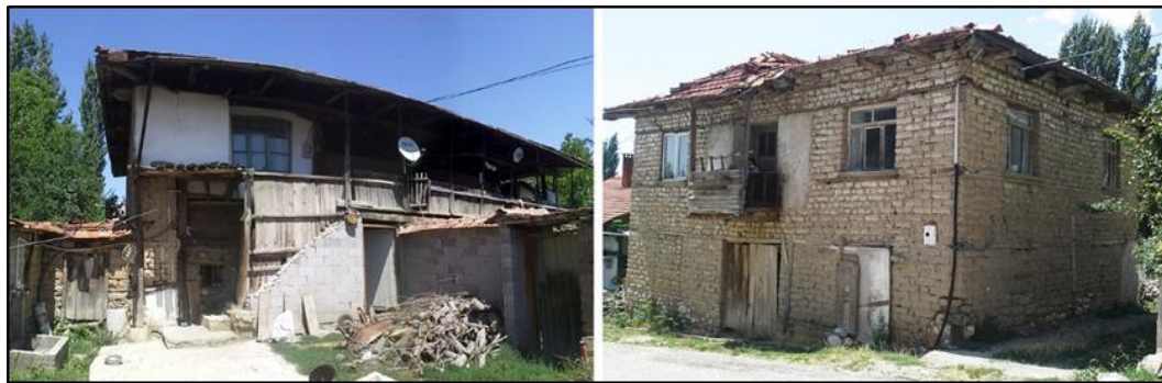
Figure 19: The early period house on the left and the late period house on the right.
