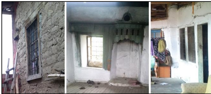
Figure 102: Windows with iron bars. Photos are taken from H13.
