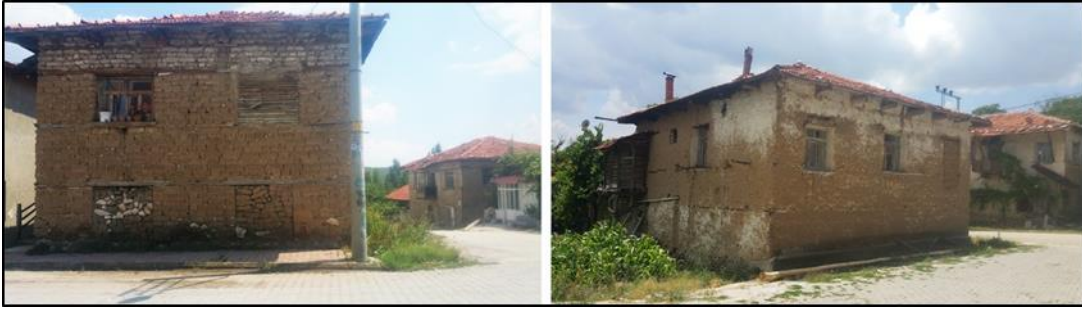
Figure 16: Street views show traditional mud brick masonry houses, located separately, in Ağlasun and the stone masonry constructed up to the sub-basement level.
