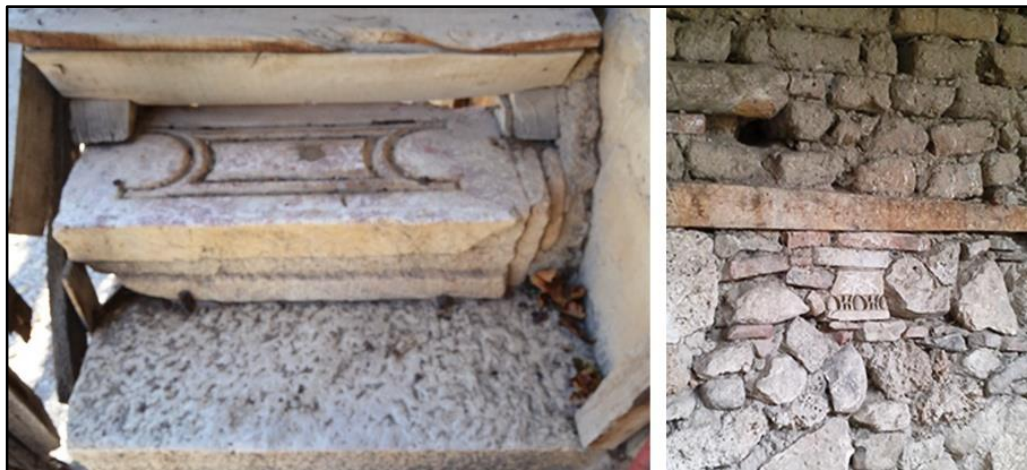
Figure 146: Spolia as a part of a staircase and the stone masonry wall. The photo on the left is from the H19 and the photo on the right is from the H13.
