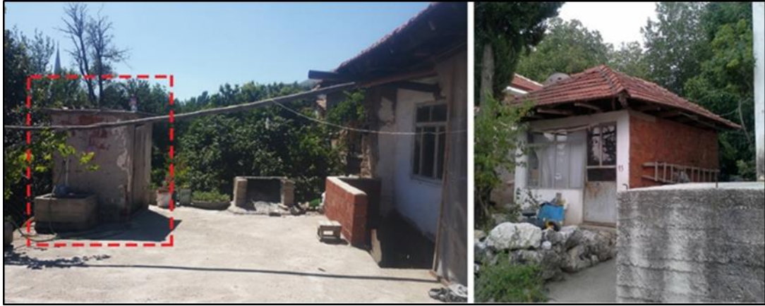
Figure 133: The photo from H2 on the left shows the toilet as a mass addition on the 'saçak'. The photo from H11 on the right shows the auxiliary building as a mass addition separately located on the same lot with the main housing.
