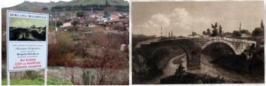
Figure 4.5 The place of Kazancı Bridge that was fallen down by the flood (ÇEKÜL (2013) An example of Urban Conservation: Bergama. retrieved from https://www.cekulvakfi.org.tr/haber/kentsel-korumada-ornek-bergama )
