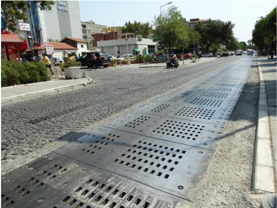
Figure 4.14 Cobblestone pavement and rain water drainage channel in Bergama (taken by the author in Bergama, 2019)
