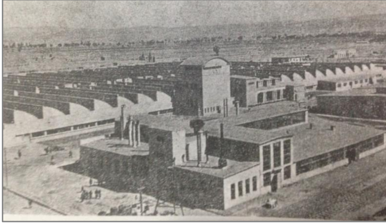
Figure 2.5. An old photo of Kayseri Sümerbank Factories, from Arkitekt-5, 1935 (Bozdoğan, 2012:142)
