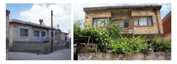
Figure 4.38. Examples for masonry walls with RC Frame slabs of new buildings
