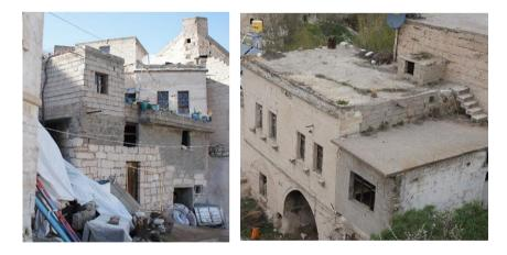
Figure 4.31. Examples for mass additions in vertical dimension
